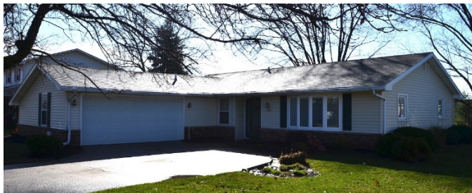
Attached accessory structure
