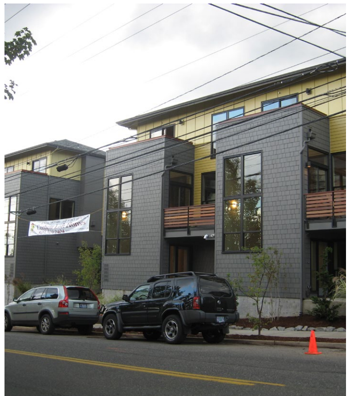
R1 zone project with lower height close to the street frontage and building mass divided into two smaller components.
