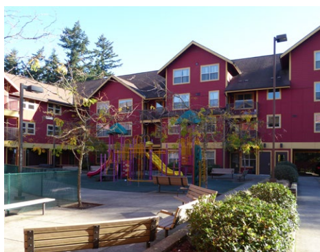
Pattern Area: Eastern Housing Type: Apartments Number of Units: 37
