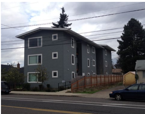
Pattern Area: Eastern Housing Type: Apartments Number of Units: 9
