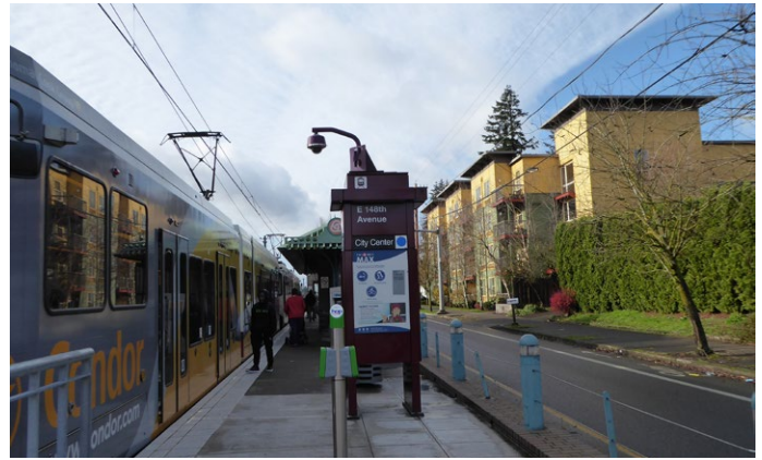
Multi-dwelling development near the 148th Avenue light rail station (RH zone)
