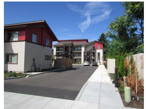
Pattern Area: Eastern Housing Type: Duplex / Apartment Number of Units: 11
