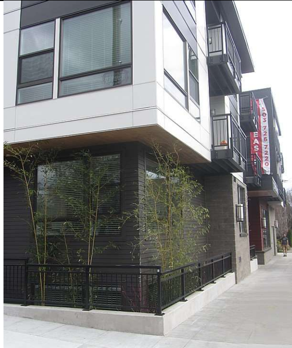
Zero setback for upper stories, and in this example, 4' for the first floor.
