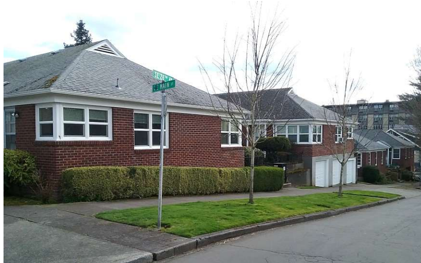
Courtyard building at zero setback. Shrubs are in ROW, behind sidewalk.
