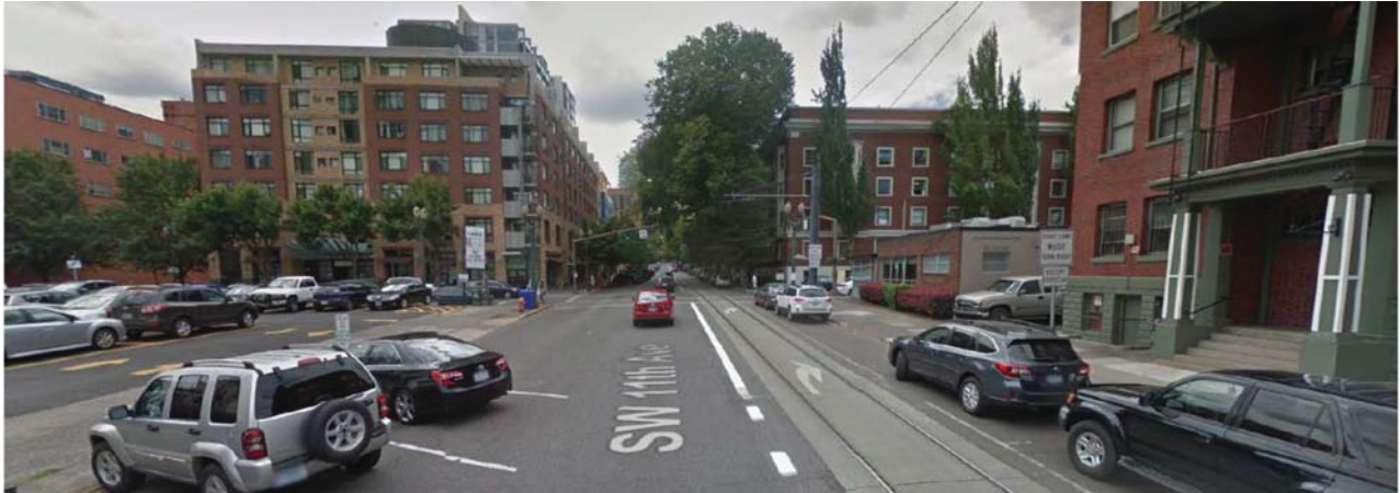
Exhibit 2. Southbound BAT lane on SW 11th Avenue from SW Stark Street to SW Clay Street, shared with Portland Streetcar alignment. This is an example of how Enhanced Transit treatments can benefit both buses and streetcars.
