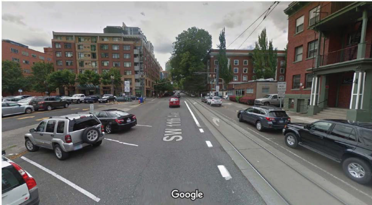
Exhibit 25. Southbound BAT lane on SW 11th Avenue from SW Start Street to SW Clay Street, shared with Portland Streetcar alignment. This is an example of how Enhanced Transit treatments can benefit both buses and Streetcar.
