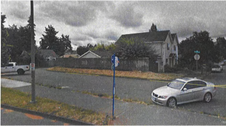
South side of Powell concrete wall
