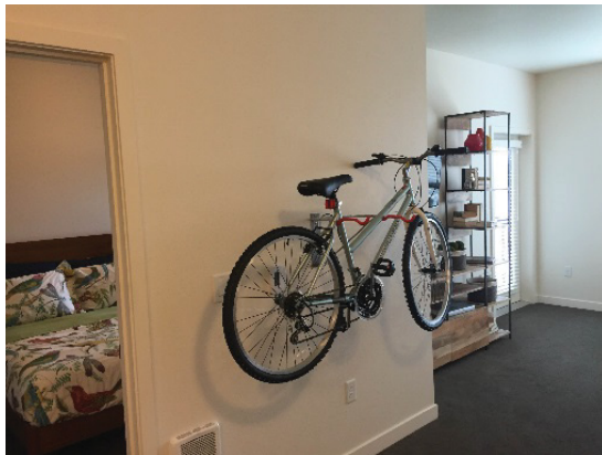
In-unit bike rack, can hold 2 bikes. 2-points of contact for each bike, but does not meet code requirements for spacing for 2 bikes.
