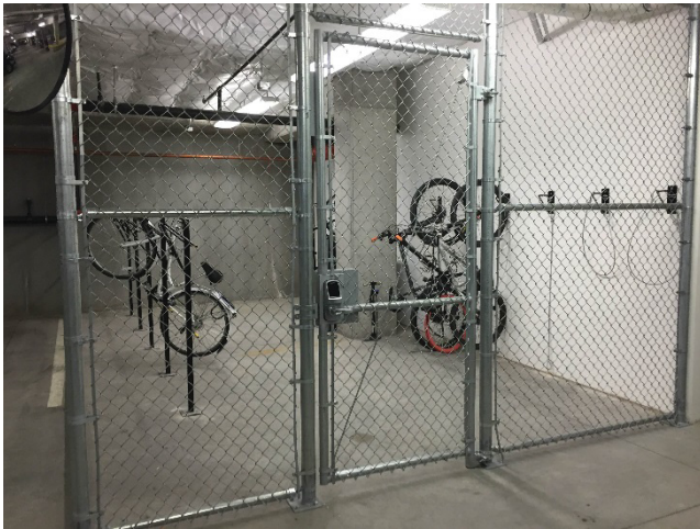
Bike cage in parking garage. Access through pin-code on door handle. All vertical parking.
