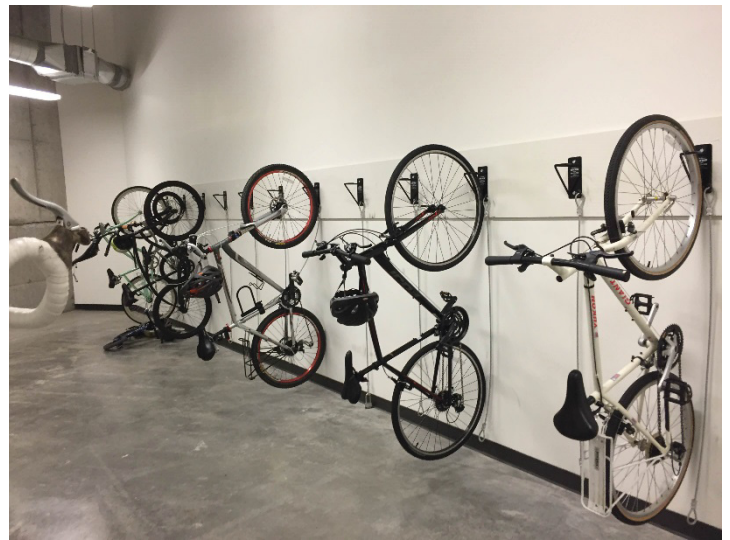
First Floor bike room, vertical cable racks.
