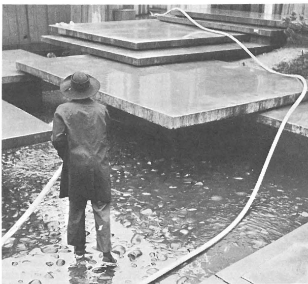
Supervising maintenance of the Auditorium Forecourt Fountain is another engineering duty. Here, maintenance mechanic washes down fountain with a fire hose.
