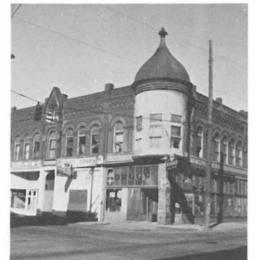
Hill building prior to demolition.
