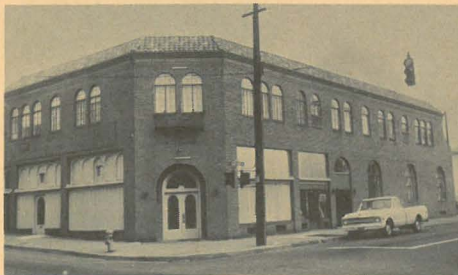
Neighborhood Development Office (NDO) #4, 4000 N. Mississippi, serving the Boise, Humboldt areas.
