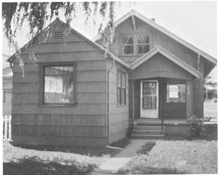
4425 N. Kerby home rehabilitated by Adams High School Home Construction Class.
