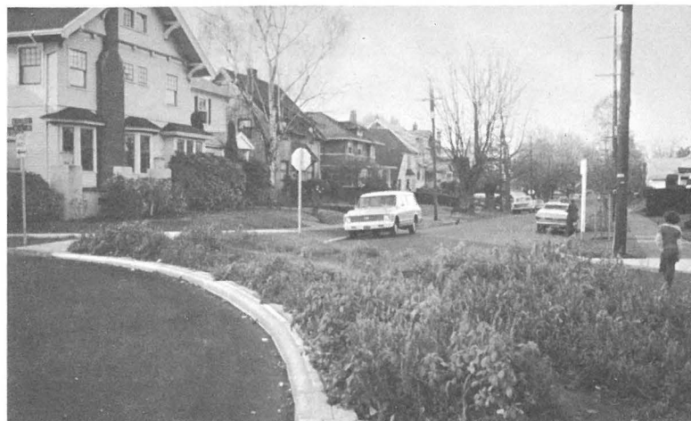
Diverter to improve residential traffic pattern is one of several traffic safety features new to the Irvington neighborhood.
