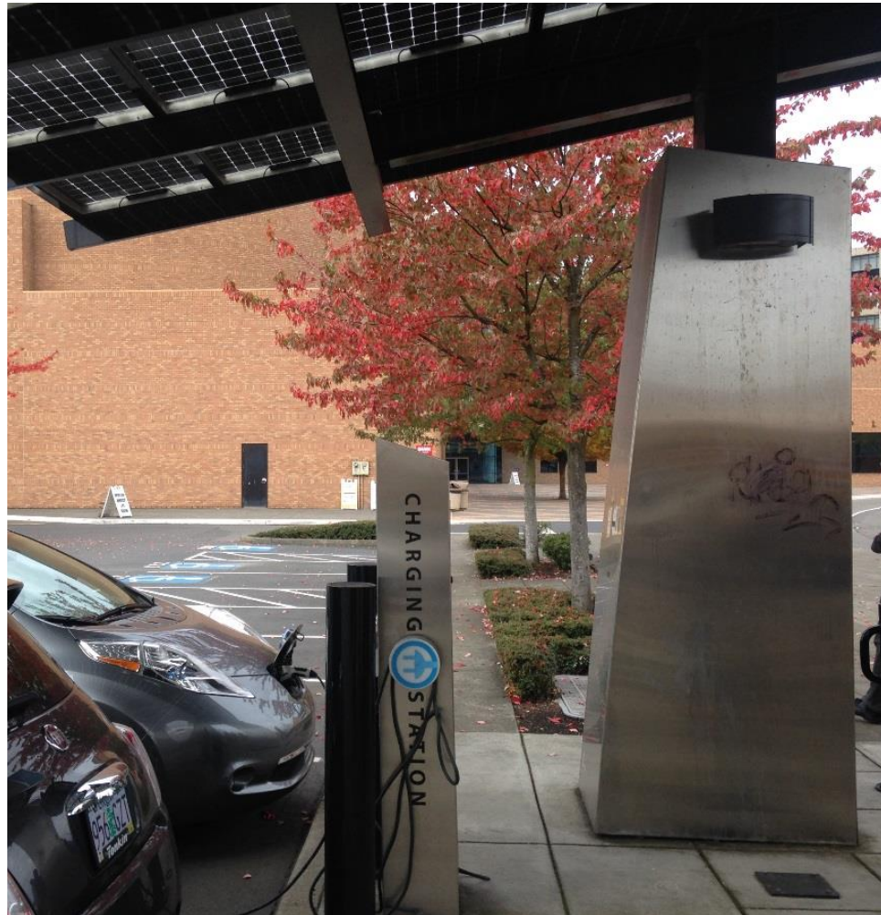
Figure 6.1.C - OMSI PV Car charging station
