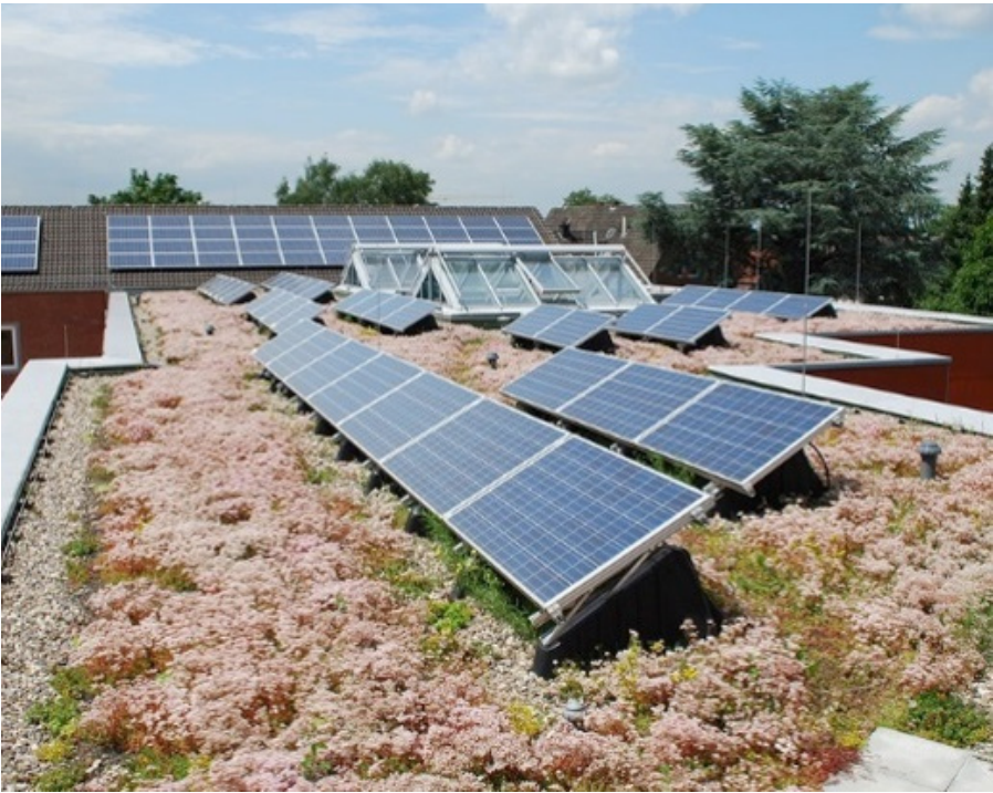
Figure 6.5.3.D - Solar photovoltaics located above a green roof, where the green roof improves the efficiency of the photovoltaic panel
