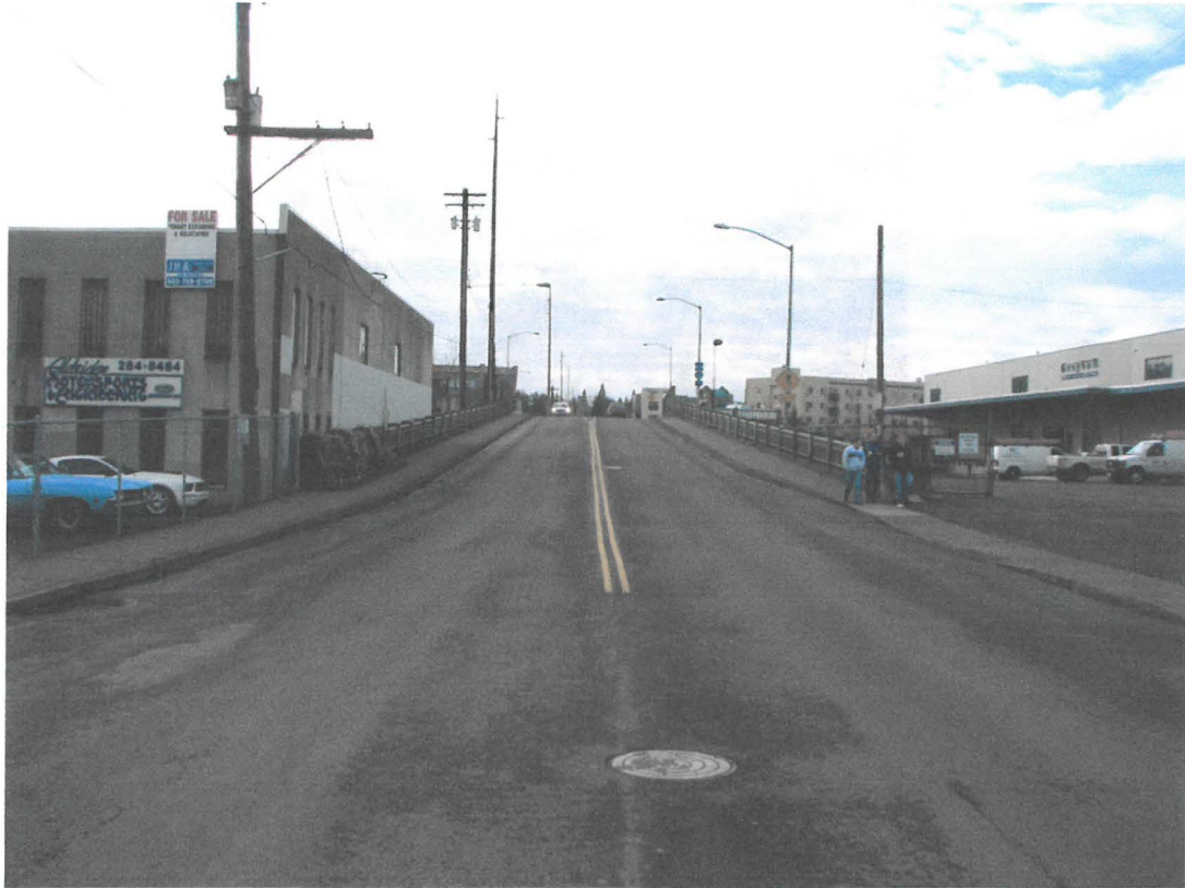
Sidewalks narrow to 3.5ft just north of 60 th Ave. MAX Station
