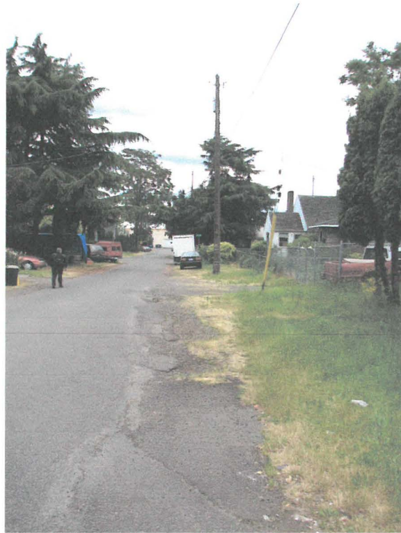
NE Hassalo and NE 60 th Ave. – Looking East
