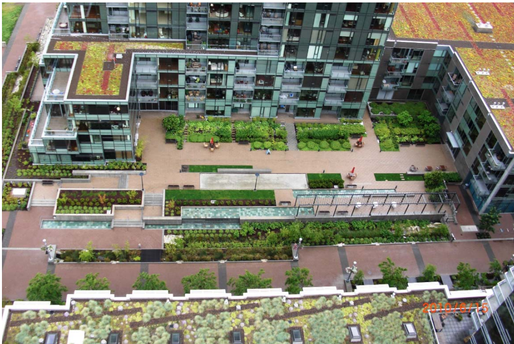
Example of a range of landscaping approaches integrated into urban development, including ecoroofs, raised landscaped areas, and stormwater planters.
