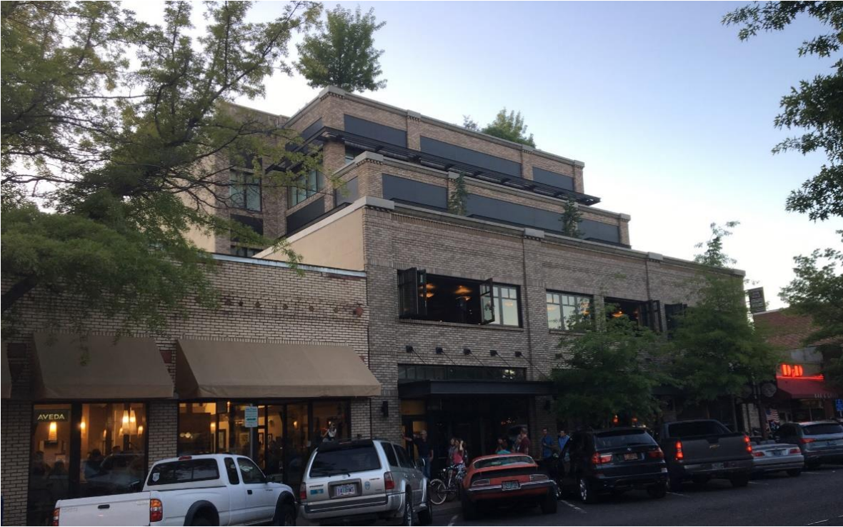
FIGURE 2 | STEPBACKS HELP COMPATIBILITY IN BEND – Not a wedding cake as BPS staff modeling shows. This is an example of good looking step backs in Bend that keep the pedestrian scale feeling of the older area while supporting more density above.
