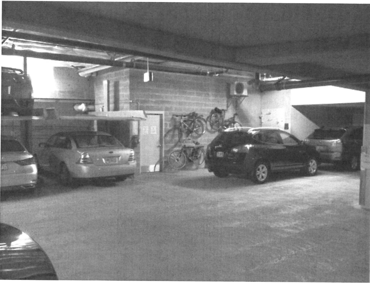
Lifts and tandem parking at The Strand condominiums in Portland. Photo by Ari Ronai-Durning.
