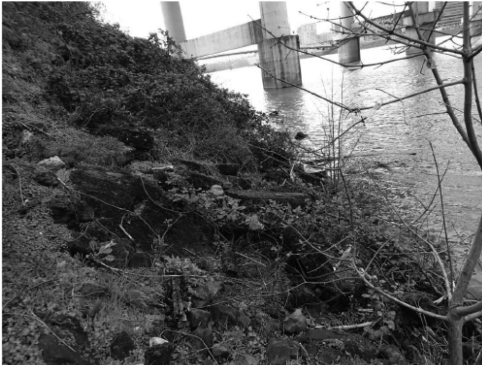
Figure 11. Blackberry and Riprap on Downstream Portion of Riverbank in Zone 3.
