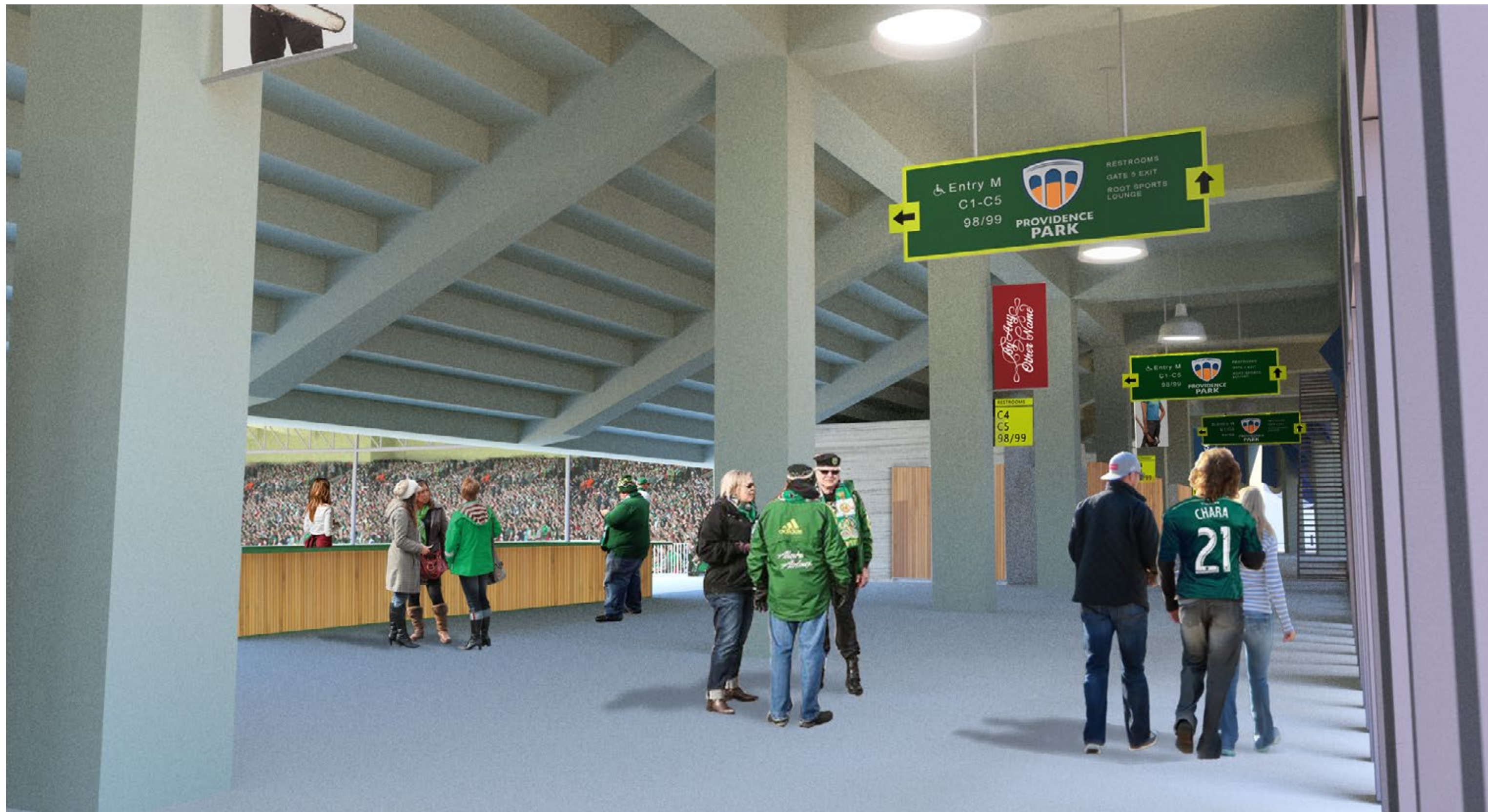
RAKER FINISH TREATMENT - EXPOSED CONCRETE
