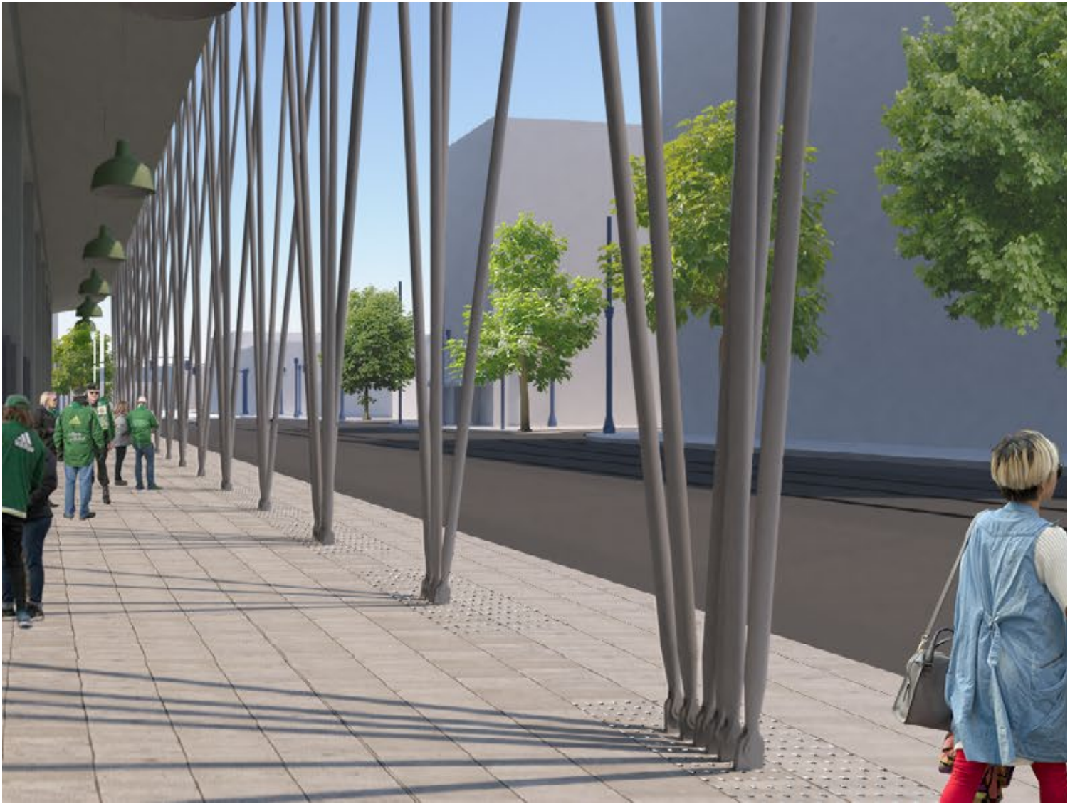
FLUSH BASE CONNECTION WITH TEXTURED CANE DETECTION
