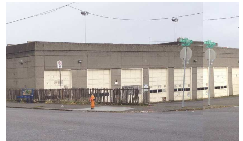
4. EXISTING STRUCTURE FROM SW CORNER
