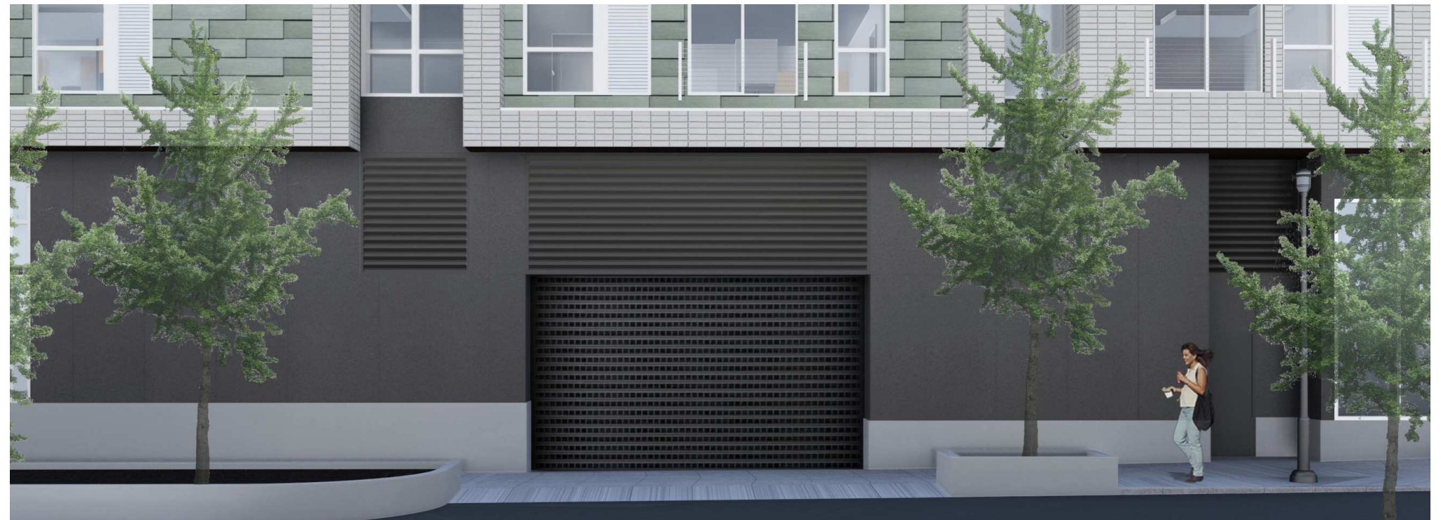
PARKING GARAGE ENTRANCE
