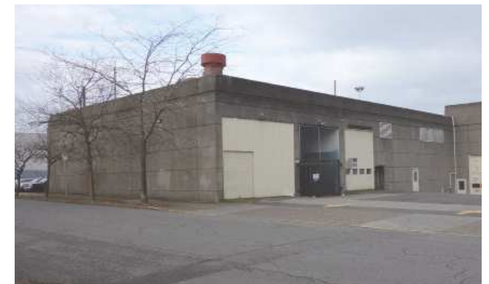
3. EXISTING STRUCTURE FROM SE CORNER
