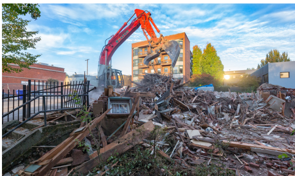
Deconstruction of an 1884 Queen Anne, ranked III on the HRI (top); demolition of a 1906 duplex in Buckman (middle); remains of the Fredrick Holman House in Goose Hollow, ranked III on the HRI (bottom).
