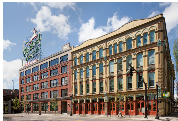
Seismic retrofit of the White Stag Block (bottom) was only feasible due to market-rate tenants and federal/local subsidy programs. Properties such as the Pittock Mansion (top) have a more difficult time funding and accomodating seismic interventions.
