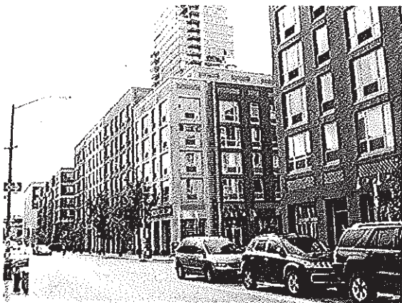
Palmer's Dock and Edge Community Apartments are the affordable housing component of the larger Northside Piers and Edge developments along the Brooklyn waterfront. Both projects, located within the Greenpoint-Williamsburg inclusionary housing designated area, received density bonuses and tax abatements from the city in exchange for providing affordable housing. New York City Department of City Planning
