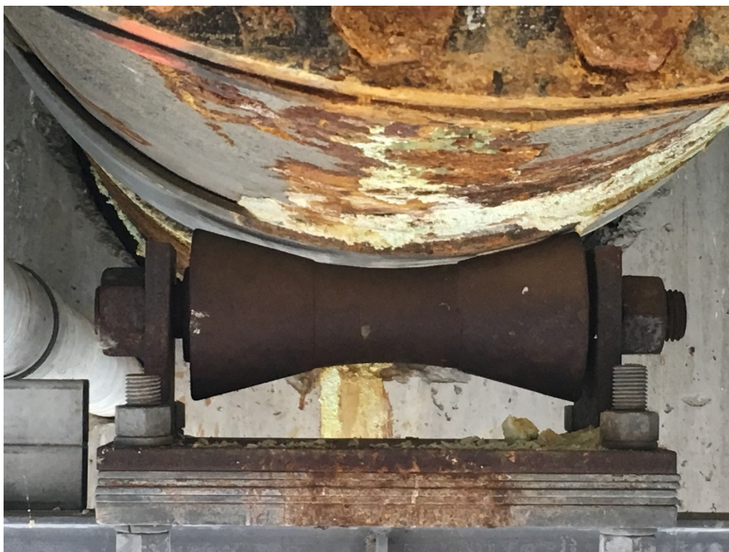
Photo 18 – Roller support at beam #13 with roller only in contact on the west side of the pipe shield.
