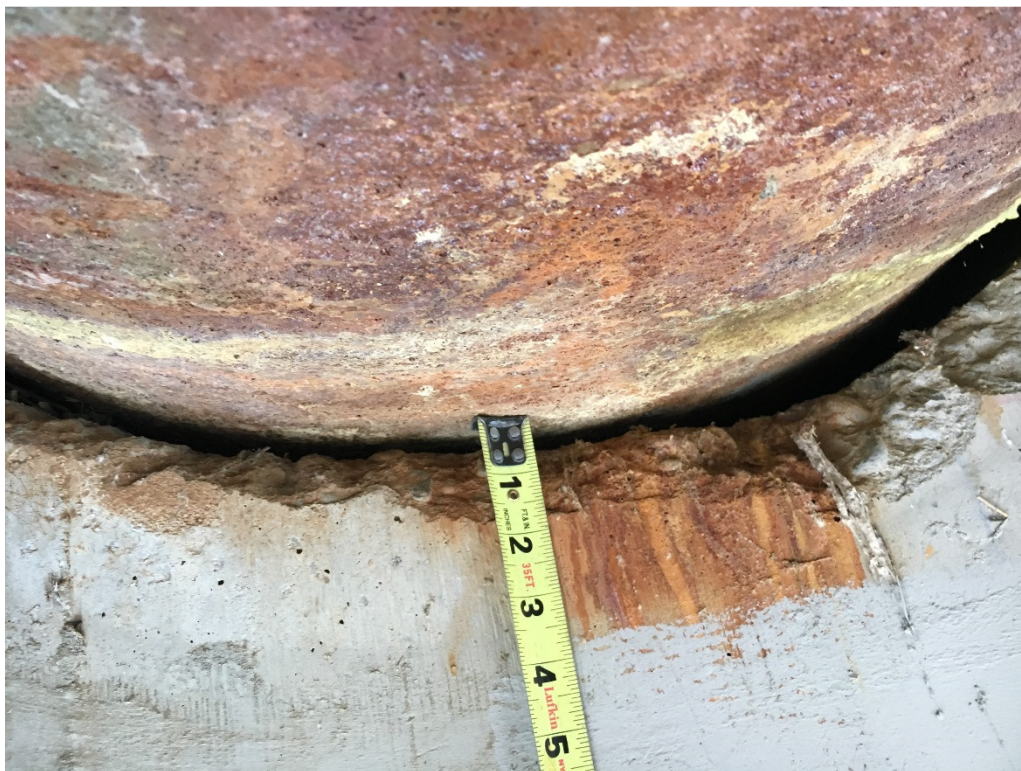
Photo 17 – Reduced clearance at bent 2 where 30-inch CIP passes through concrete diaphragm.
