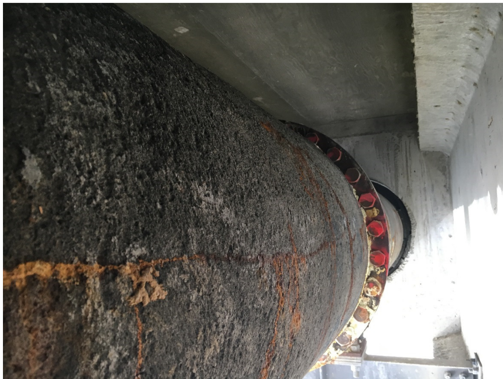
Photo 14 – Longitudinal cracking and minor staining on the west side of the pipe at approximate Sta. 23+50.
