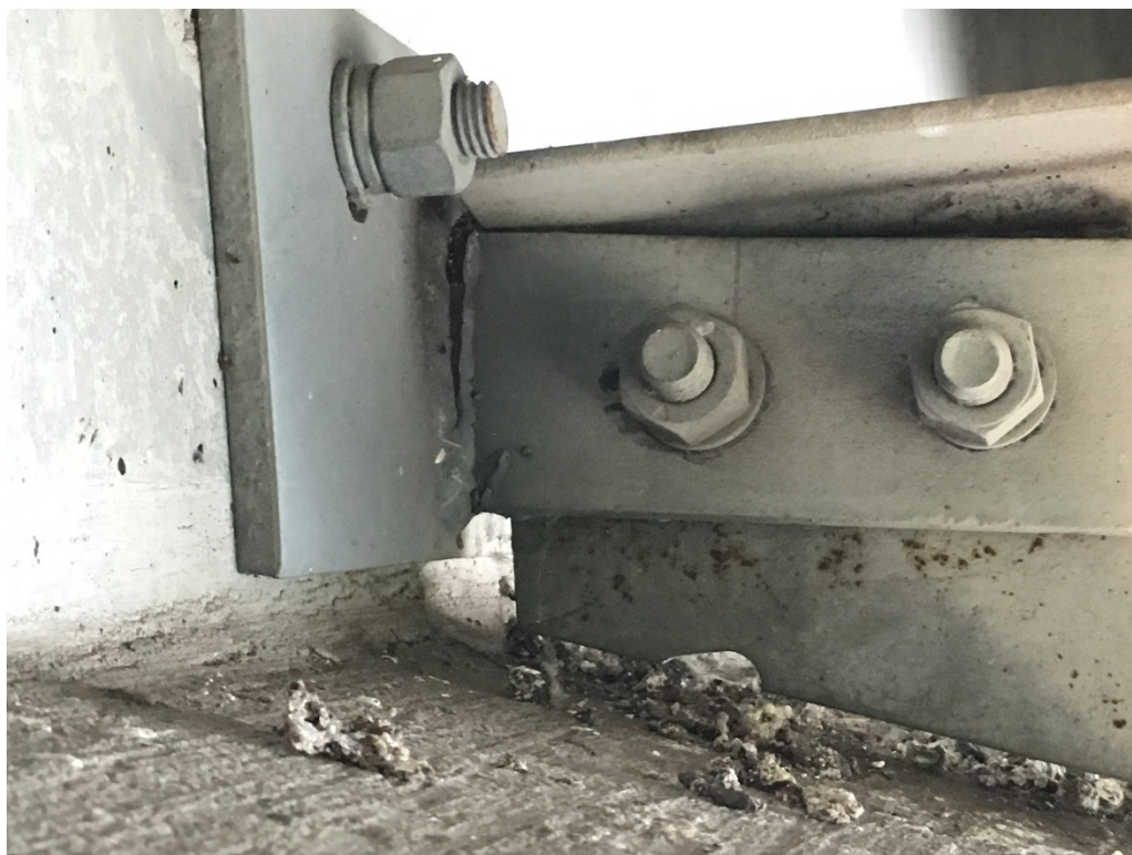
Photo 10 – Failed weld on support beam #5
