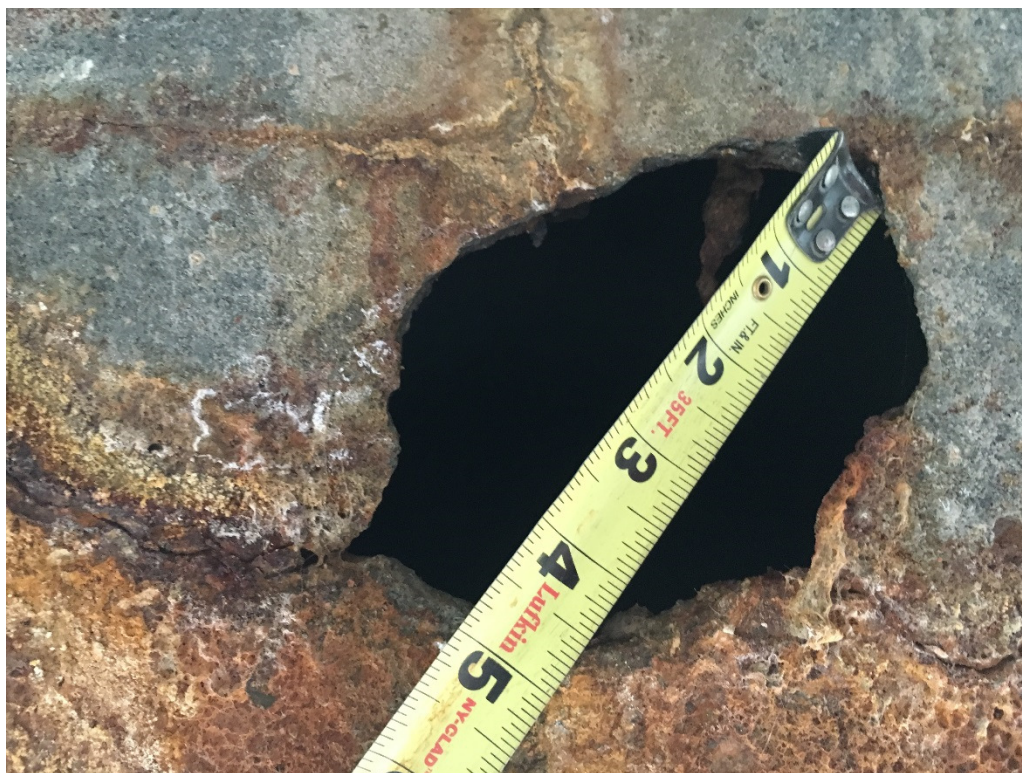
Photo 4 – Enlarged hole on west side of CCP between roller supports #8 and #9.
