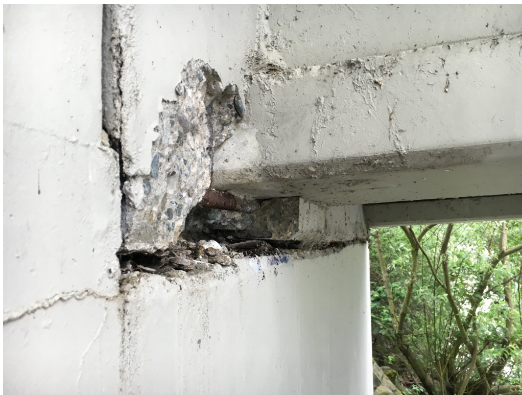
Photo 12 – Cracked concrete under east girder at bent 1.
