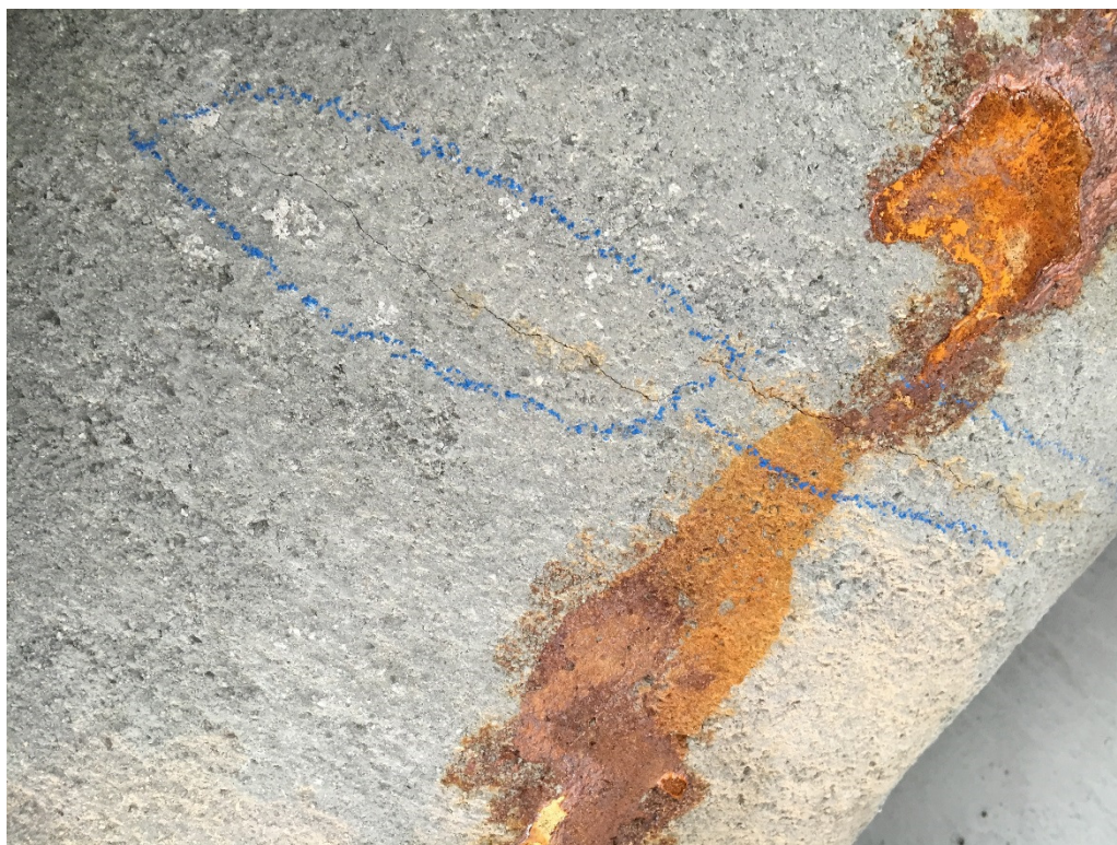
Photo 15 – Hoop cracking on the bottom of the pipe at approximate Sta. 23.50.
