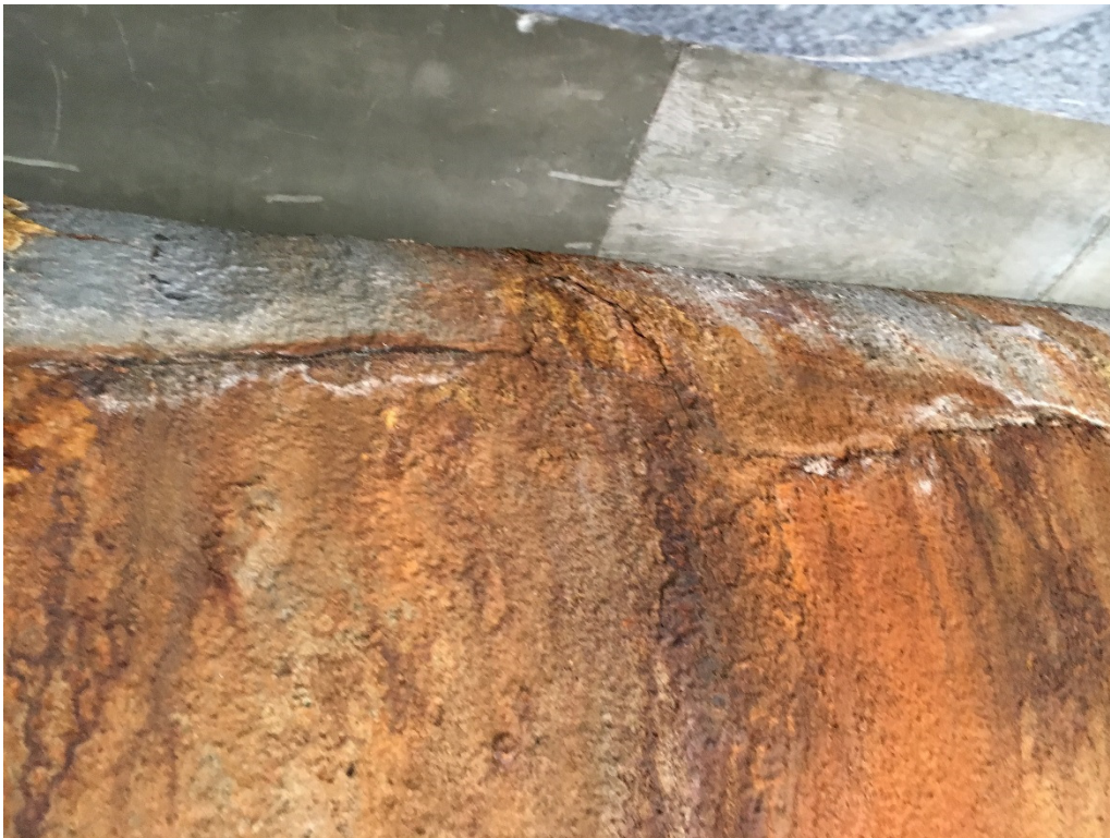
Photo 3 – Horizontal cracking and areas of concrete beginning to delaminate on the east side of CCP near bent 2
