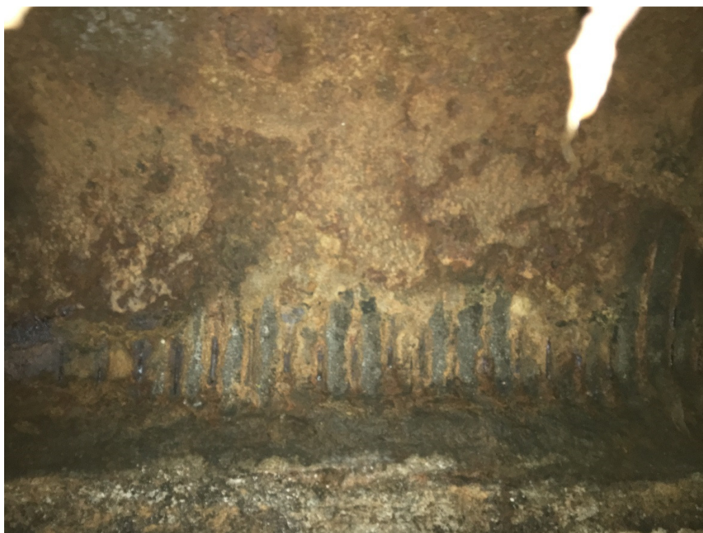
Photo 5 – Exposed exterior spiral reinforcement.
