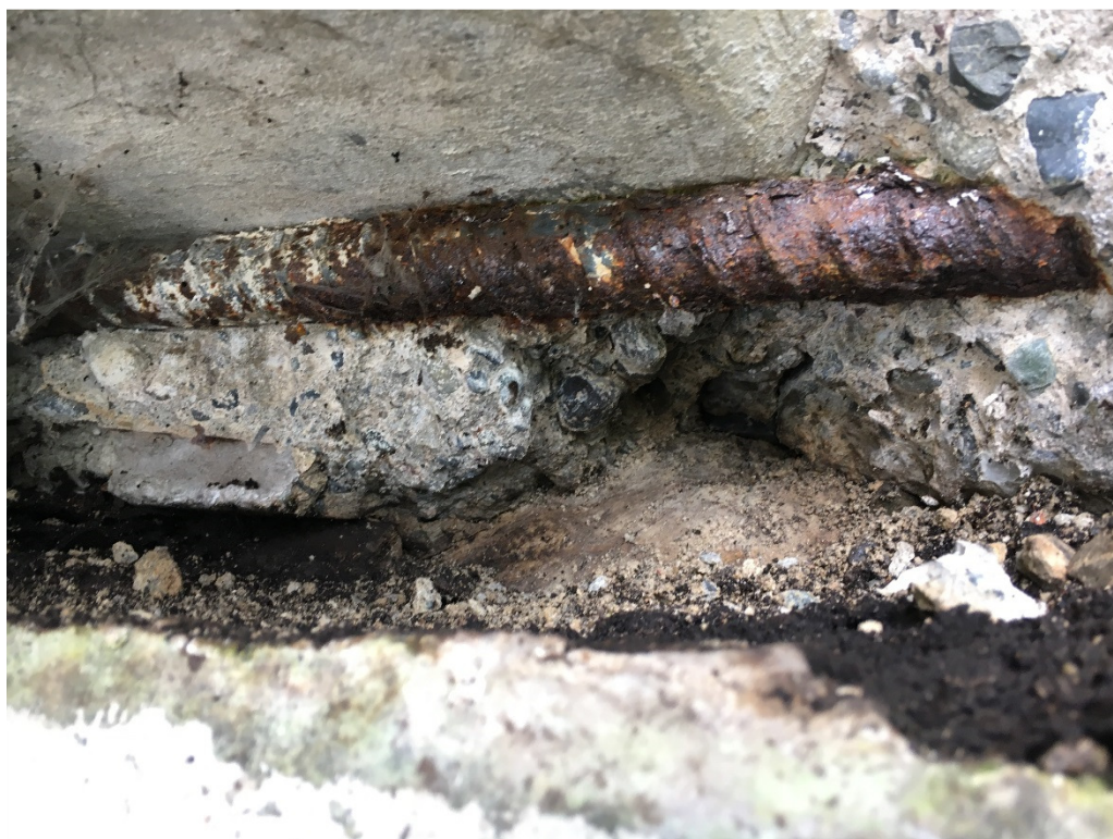
Photo 13 – Exposed and rusted diaphragm reinforcement under west girder at bent 1.
