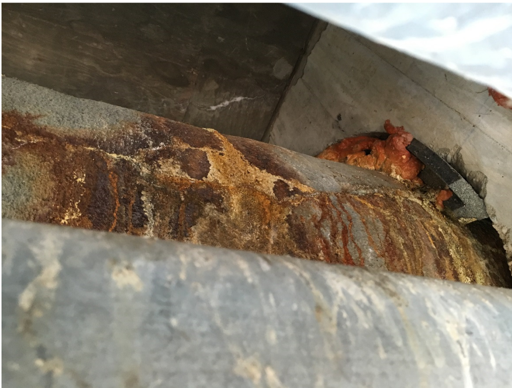
Photo 1 – Insulation and spray foam around CCP at bent 2.
