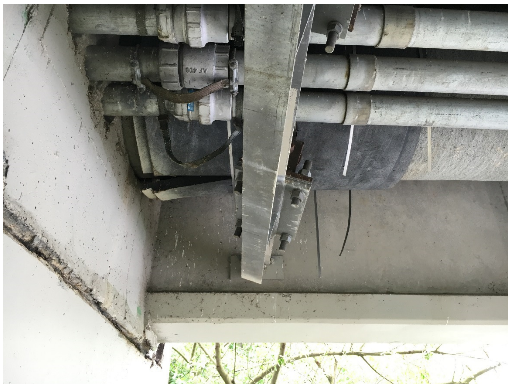
Photo 8 – Rotated pipe support beam at roller #1
