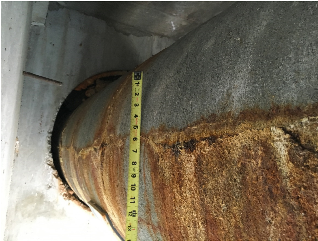
Photo 2 – Horizontal cracking on west side of CCP near bent 2.
