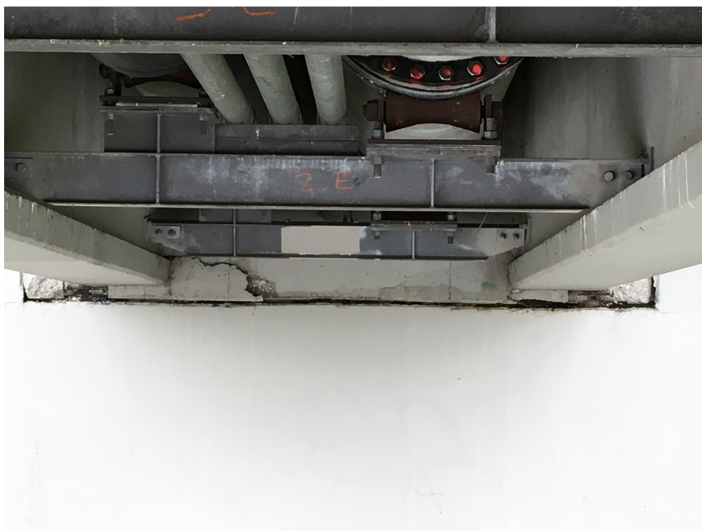
Photo 11 – Cracked concrete under girders at bent 1.
