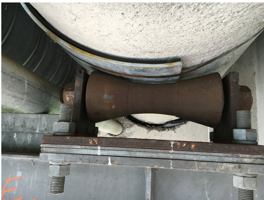
Photo 7 – Rotated pipe shield at support #4.
