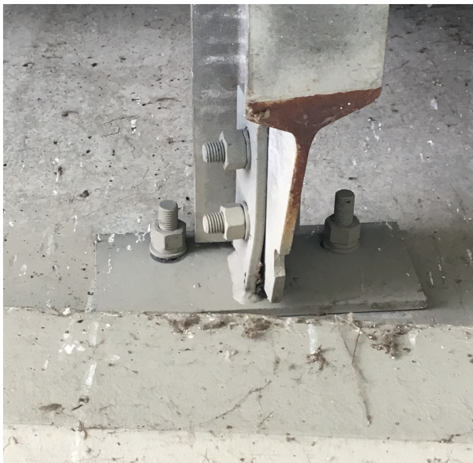
Photo 9 – Rotated girder to support beam connection plate at
