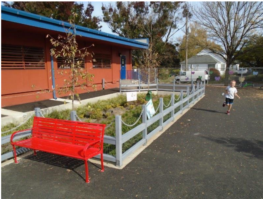
Figure 23 FY 2016 Example Retrofit #2
