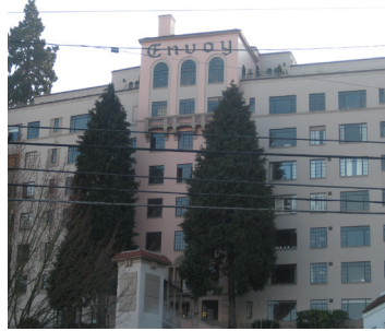
Address: The Envoy Existing FAR: - Height: 100' Lot Size: 38,000 sf Contributing Building
