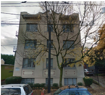
Address: 2060 NW Lovejoy St. Existing FAR: 2.619127 Height: 38.01' Lot Size: 5000 sf Contributing Building
