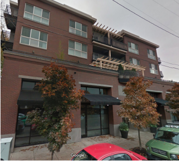
Address: 210 NW 20th Ave Existing FAR: 1.471825 Height: 45' Lot Size: 10,500 sf Non-Contributing Building
