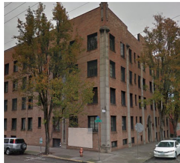
Address: 1983 NW Flanders St. Existing FAR: 1.359173 Height: 55' Lot Size: 10,000 sf Contributing Building
