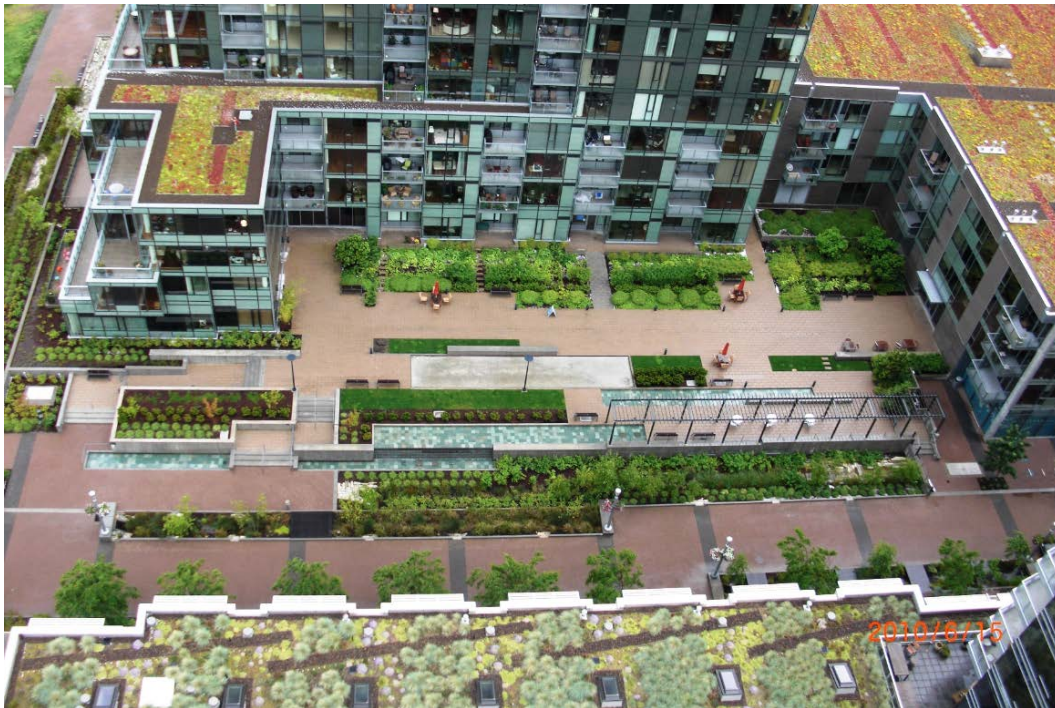
Example of a range of landscaping approaches integrated into urban development, including ecorooftops, raised landscaped areas, and stormwater planters.
