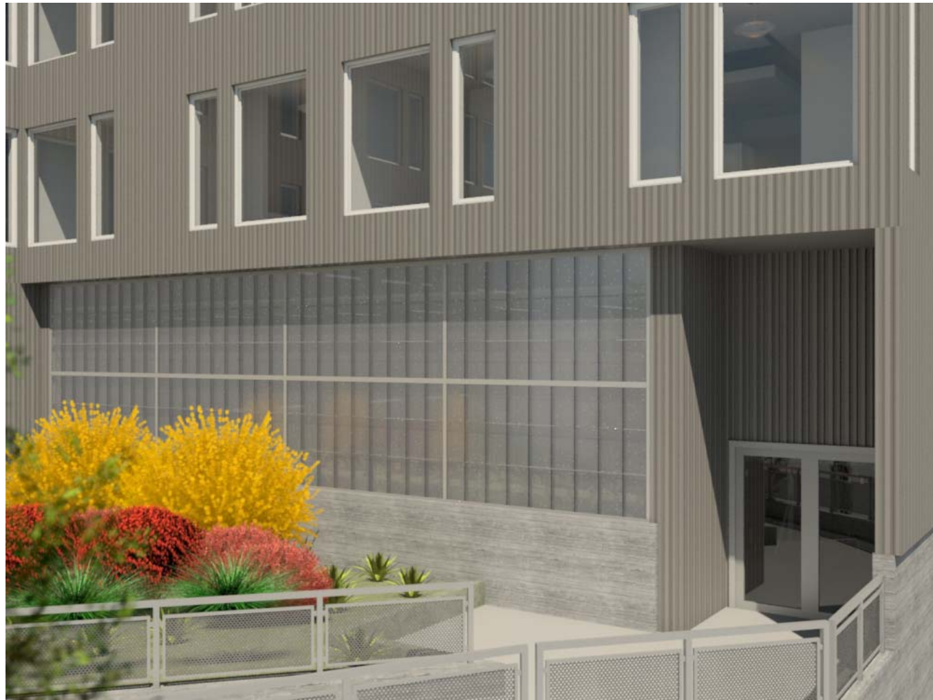
Bike Room Structure - Kalwall Clad
