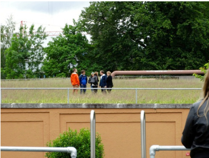
Figure 5 Ecoroof on water storage building Zurich constructed 1914 still intact.
