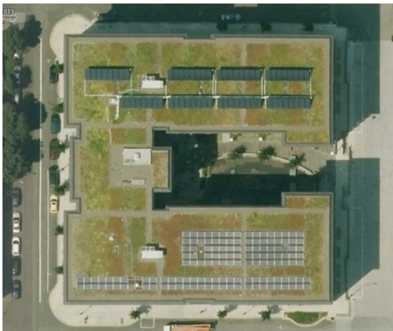
Figure 1. Ramona Apartments with solar hot water panels and PV panels installed 2011
