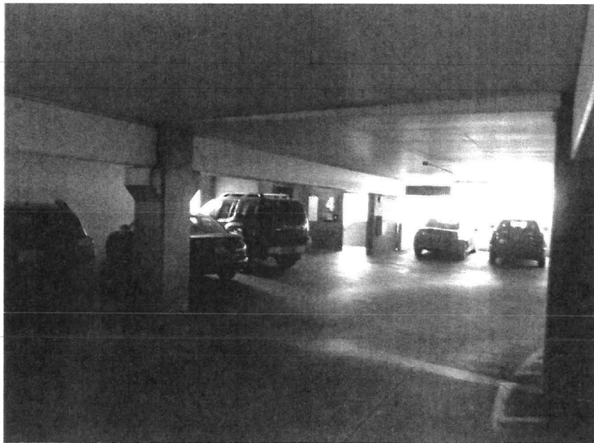
Figure 9, Concrete framing system in the 4 th floor
