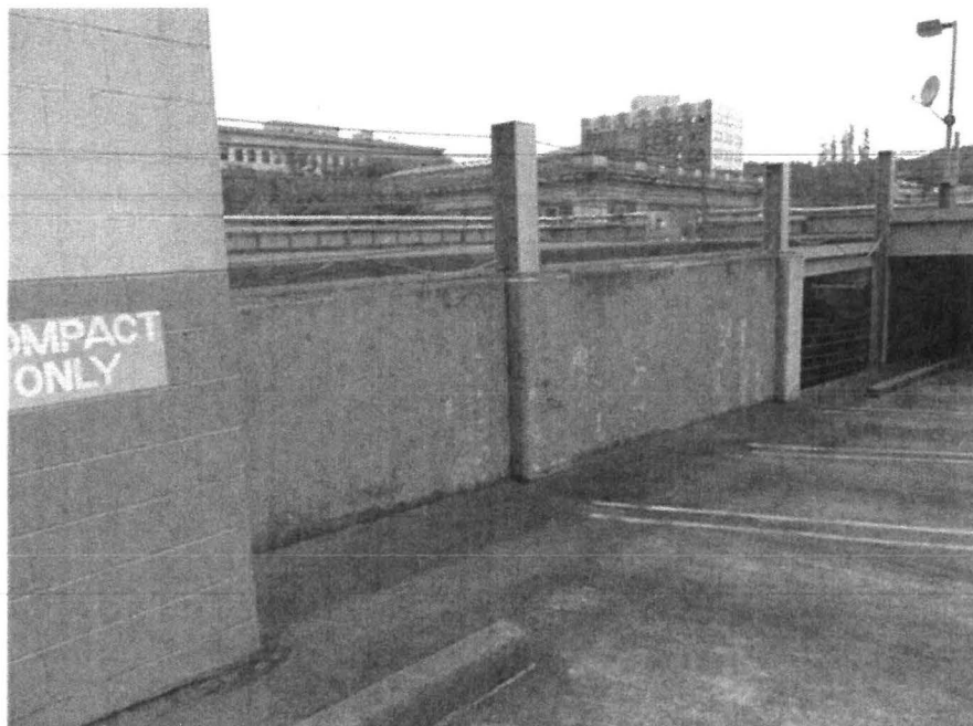
Figure 7, Shear walls in the E-W direction
