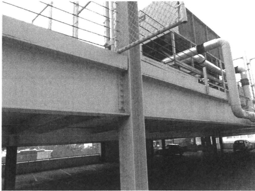
Figure 2, Steel framing in the upper floors
