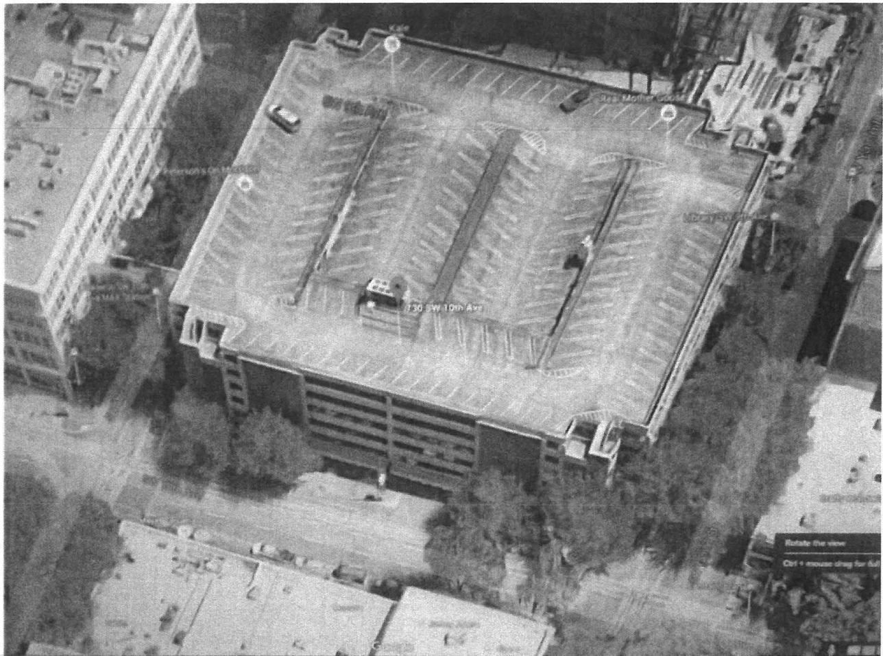
Figure 1, Overview of the Garage Building (Source: Google)
