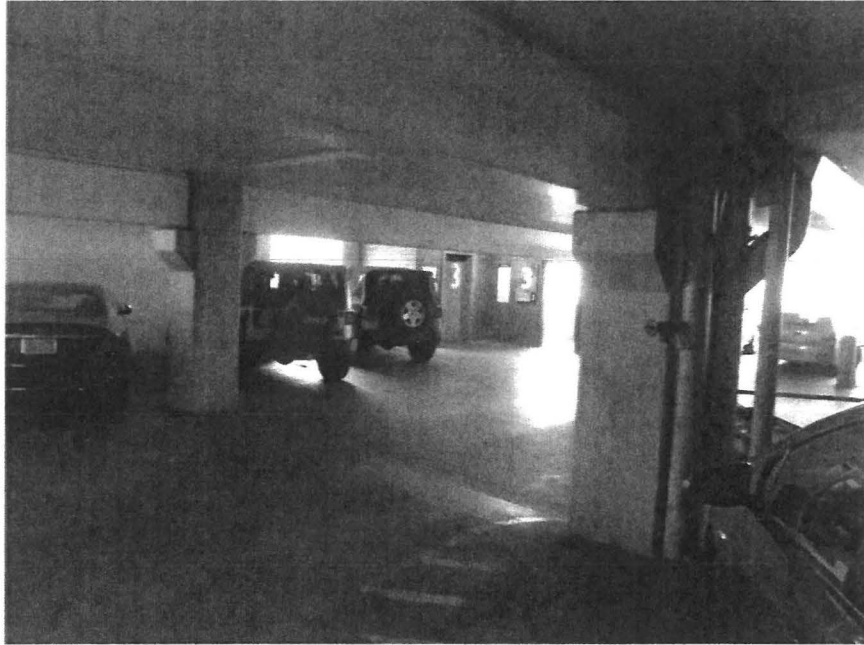
Figure 10, Concrete framing system in the 3 rd floor
