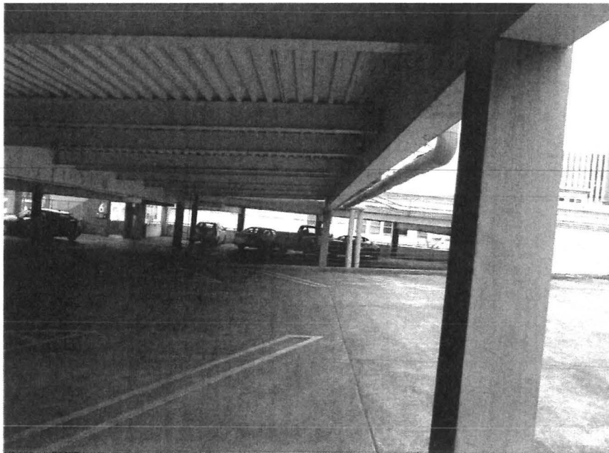
Figure 3, Composite floor construction, upper floors
