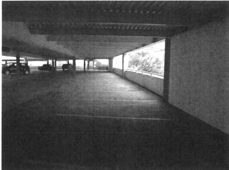
Figure 6, Shear walls in the N-S direction
