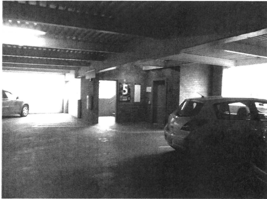
Figure 8, Framing system in the 5 th floor
