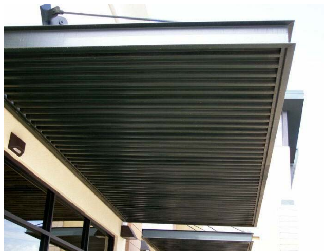
EXAMPLE OF PROPOSED CANOPY STRUCTURE
