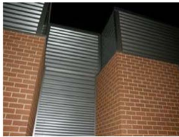
BRICK TO METAL EXAMPLE OF SIDING TRANSITION
