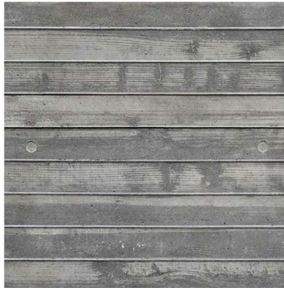
1 BOARDFORM CAST-IN-PLACE CONCRETE 1X6, ROUGH-SAWN CEDAR BOARDS, STAGGERED ENDS
