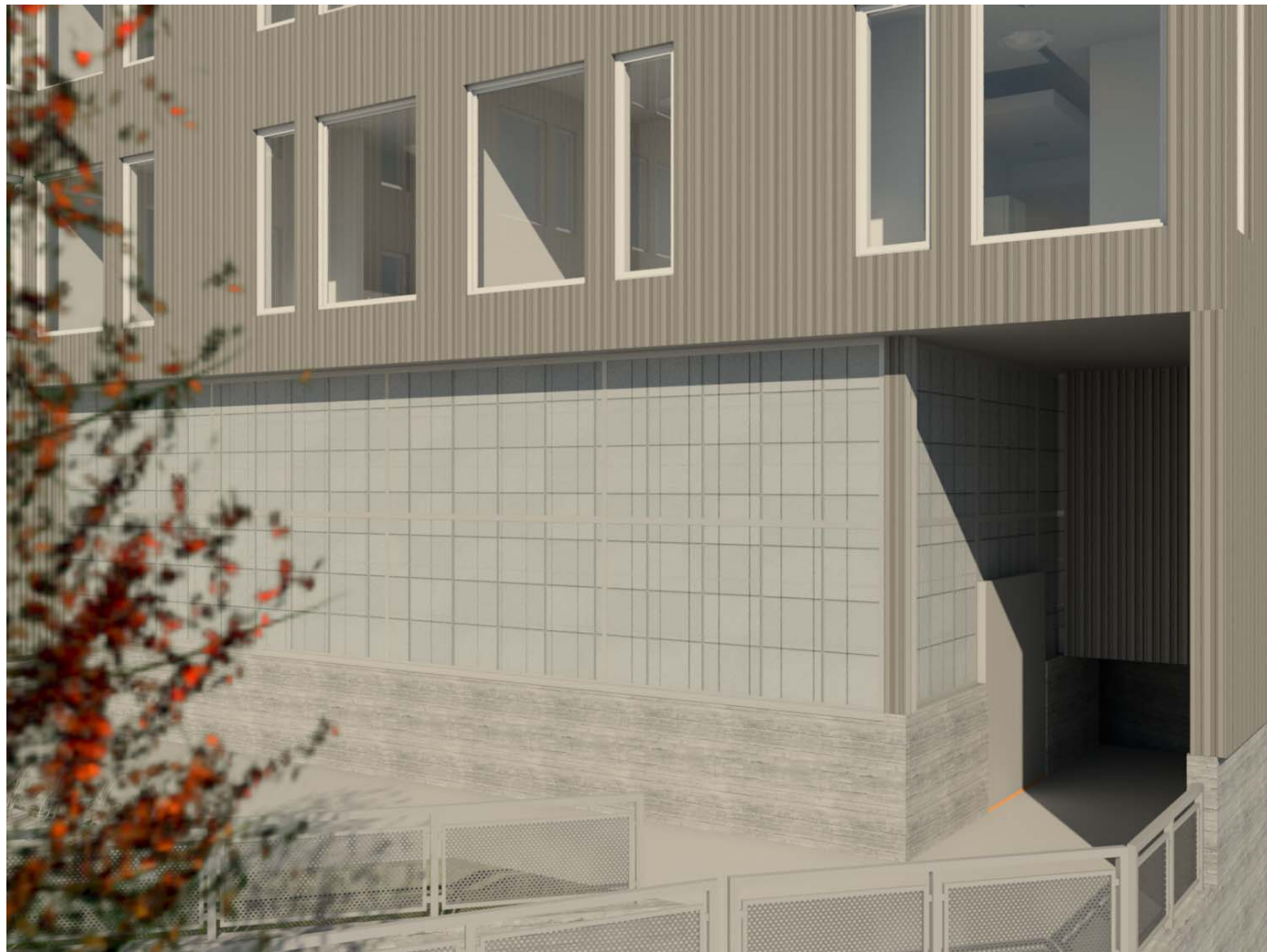
Bike Room Structure - Kalwall Clad
