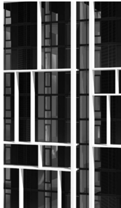
NORTH AND SOUTH FACADE
