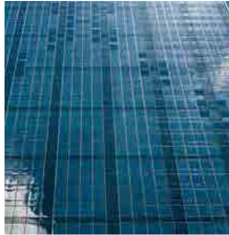
DARK GREY WINDOW-WALL WITH BACK-PAINTED GLASS PANELS
