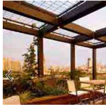
D - Overhead structure
