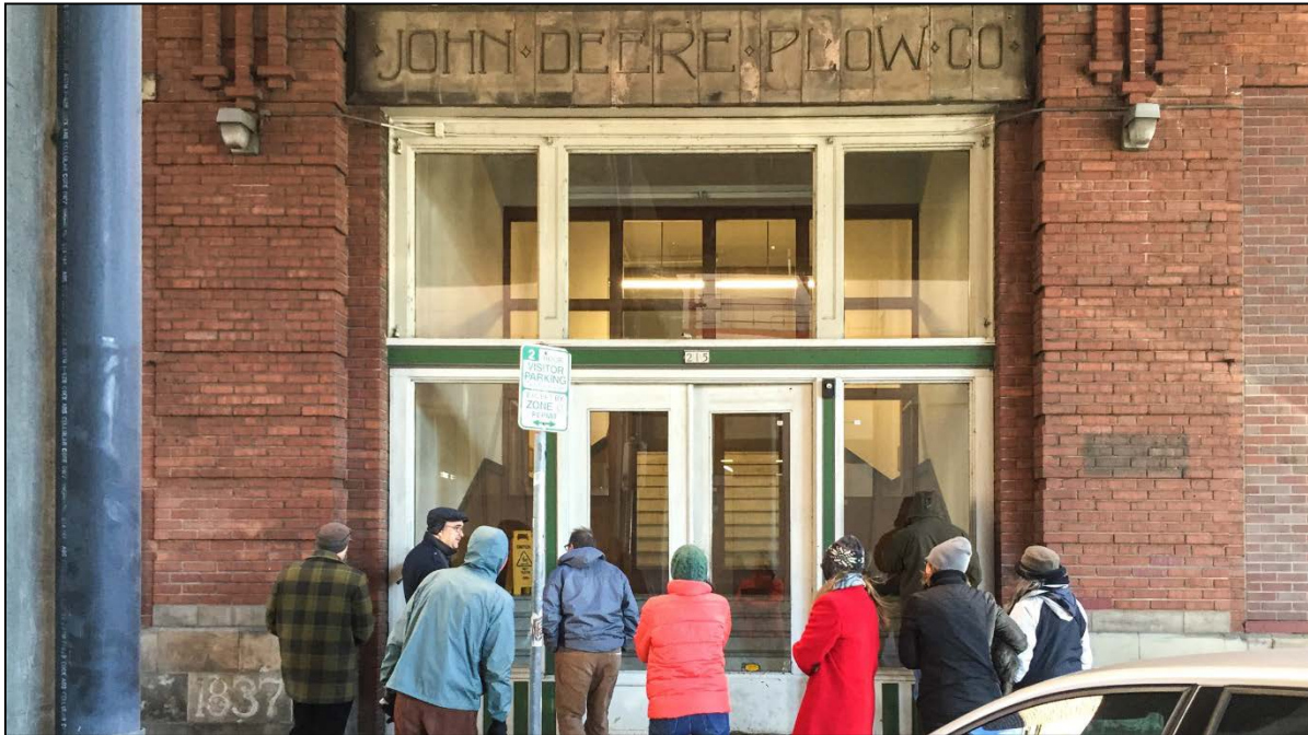
Former John Deere Headquarters, now Portland Storage building under the Morrison Bridge viaduct.
