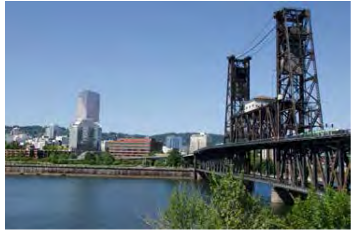
View from mid-ramp on the bike/ped path south of Steel Bridge
