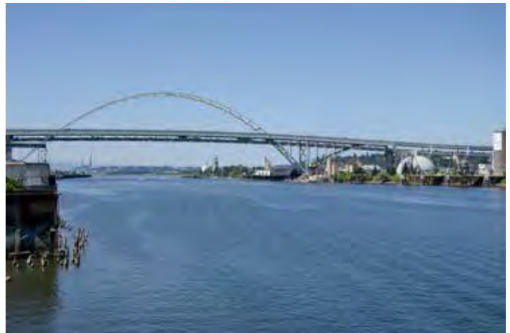
The Fremont Bridge from the Greenway Trail (west)
