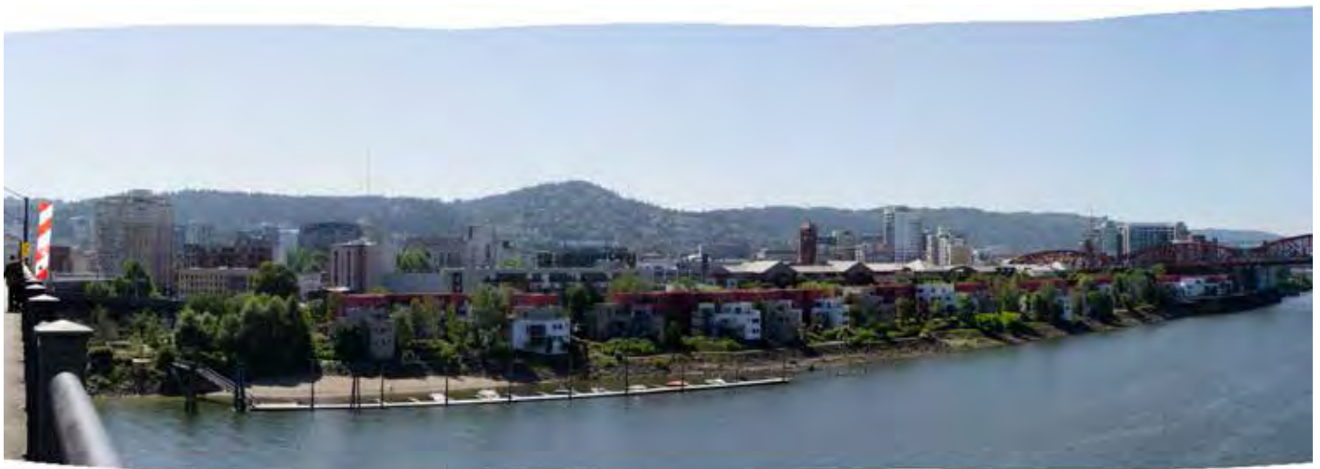
View from Steel Bridge north side east of center
