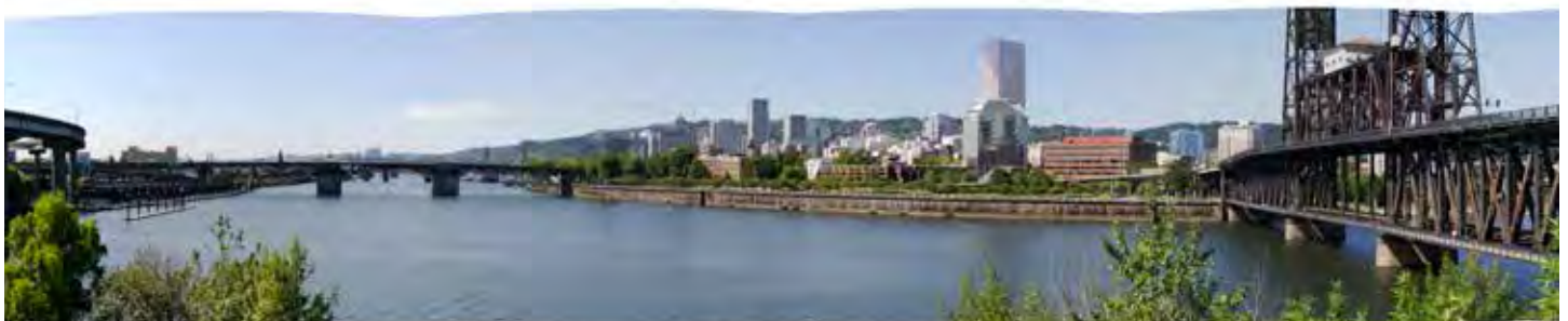
View from mid-ramp on the bike/ped path south of Steel Bridge
