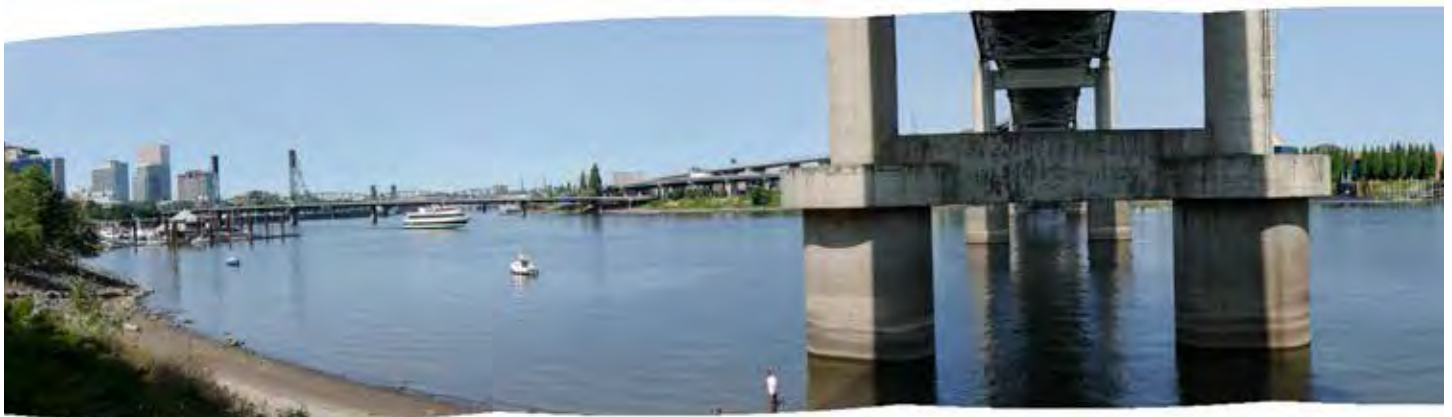
View from Greenway Trail under Marquam Bridge
