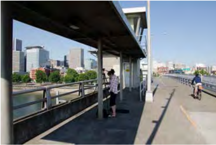
Viewpoint on Morrison Bridge south side east bump-out
