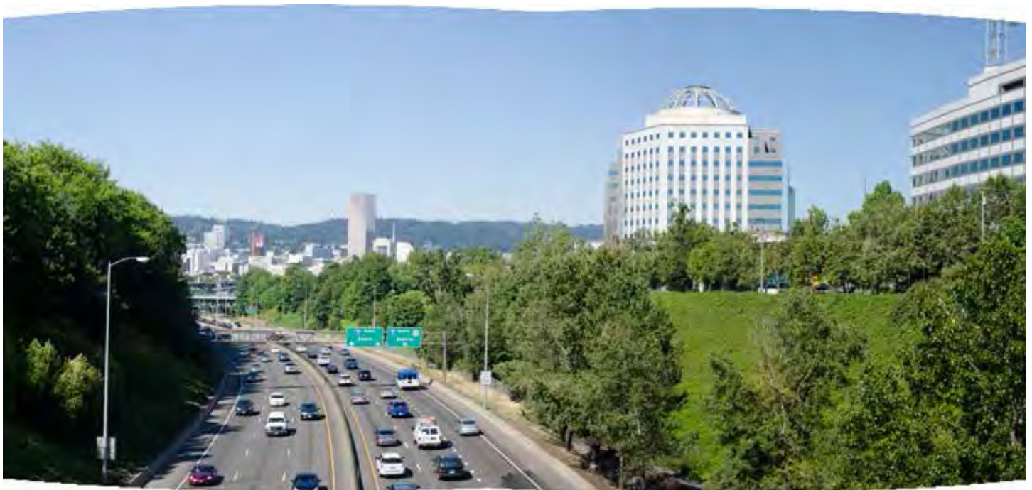
View from NE 12th Avenue and Interstate 84 overpass
