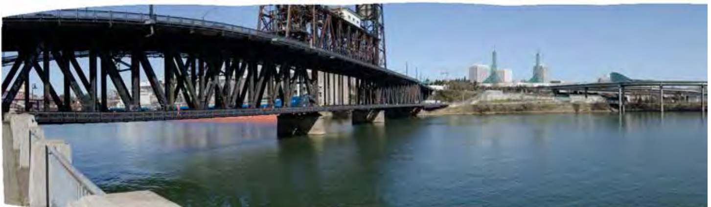
View from Greenway Trail south of Steel Bridge
