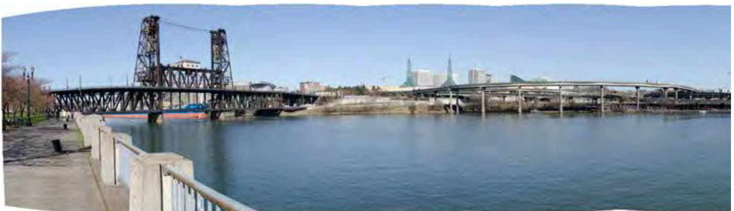
View from Greenway Trail West at stairs near NW Everett Street
