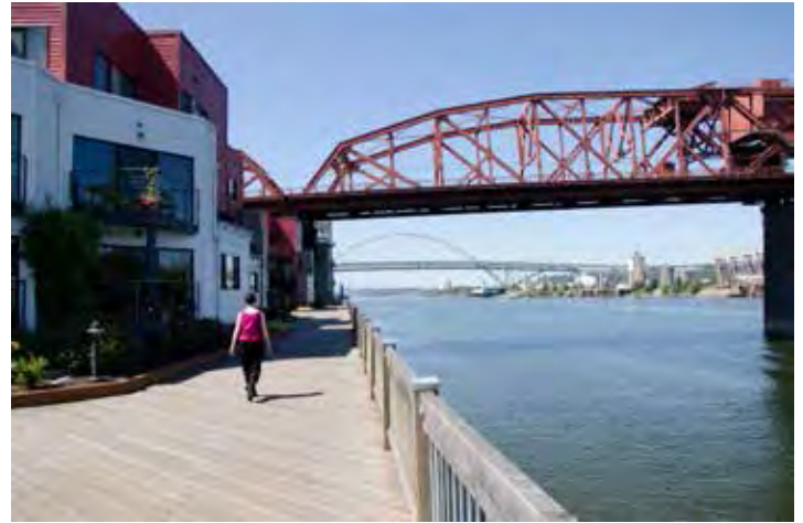
View from Greenway Trail just south of Broadway Bridge
