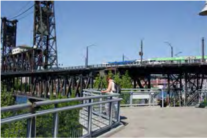
Viewpoint mid-ramp on the bike/ped path south of Steel Bridge
