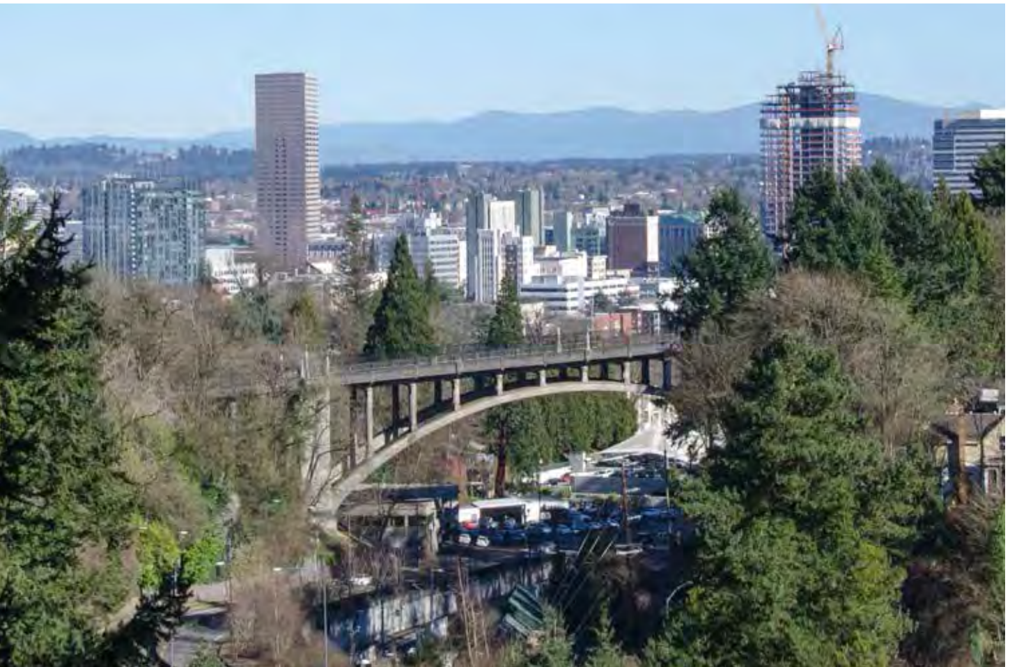
Vista Avenue Viaduct from SW Sherwood Boulevard
