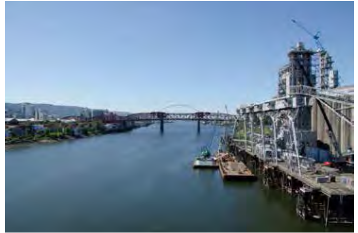
View from Steel Bridge north side east of center
