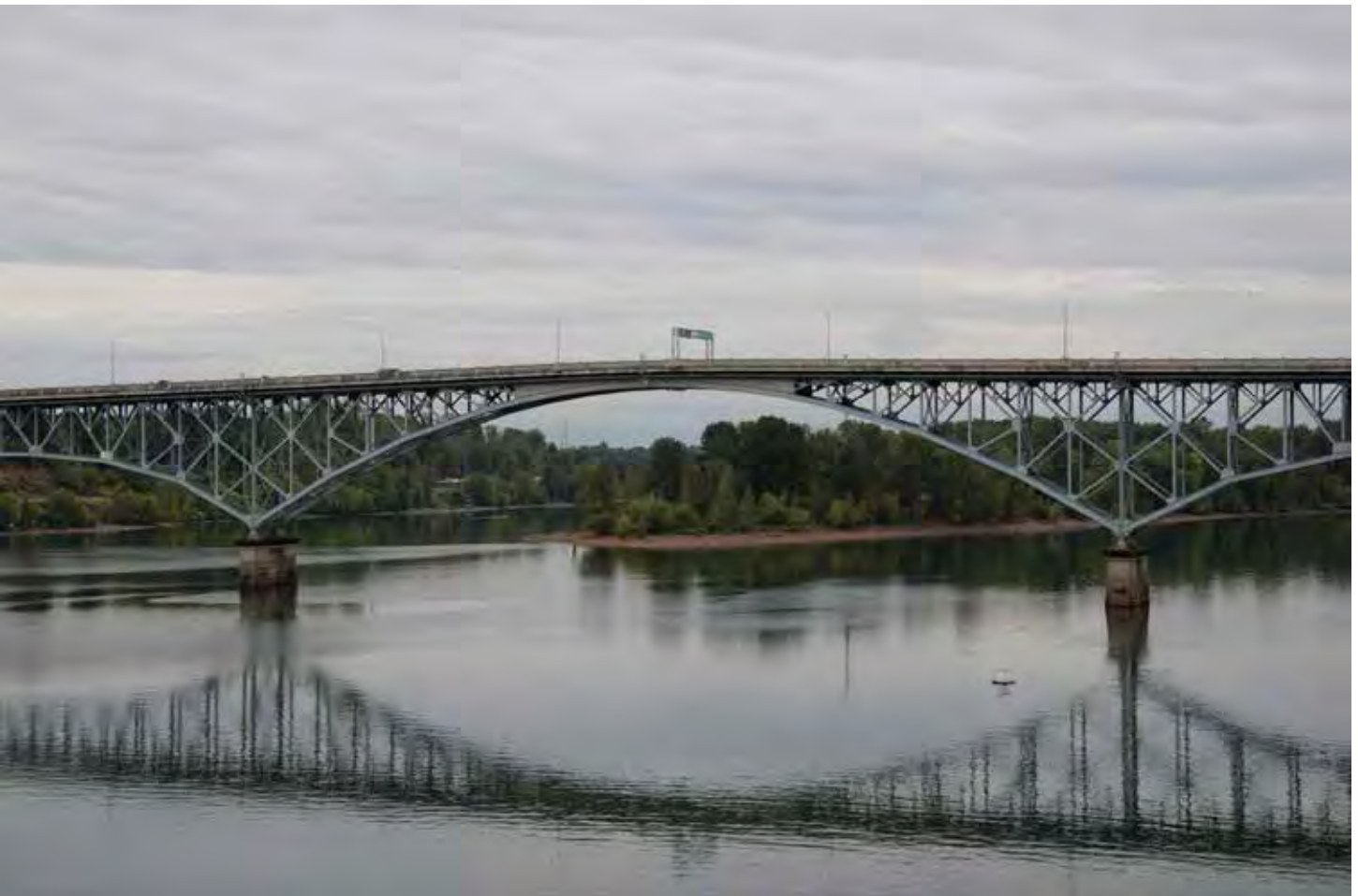
The Ross Island Bridge from Tilikum Crossing
