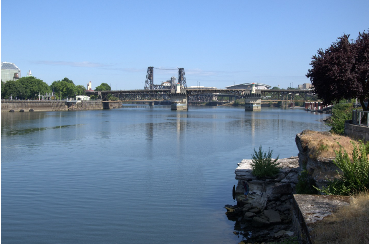
View of Willamette River as the primary focal feature, with the Steel Bridge as a contributing feature.
