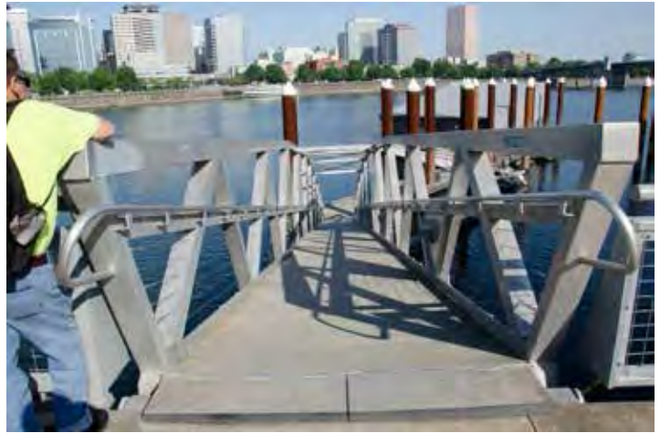
Entrance to Madison Dock
