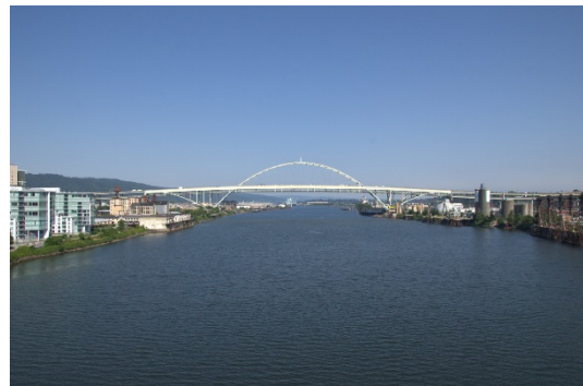
Fremont Bridge as seen from the Broadway Bridge.
