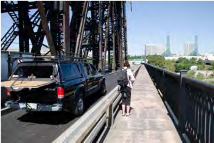
Viewpoint on Steel Bridge upper deck, south side center
