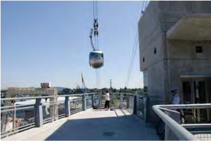
Viewpoint at SW Gibbs Street pedestrian bridge
