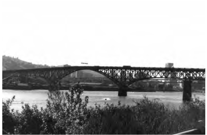
The Ross Island Bridge from Springwater Corridor circa 1988
