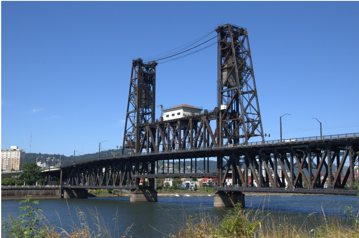
View of Steel Bridge.
