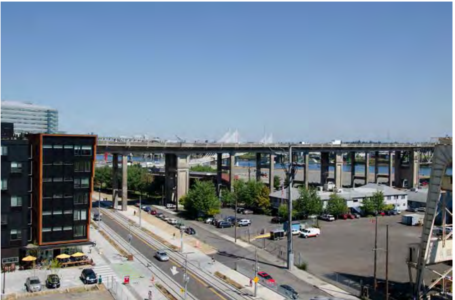
View from SW Gibbs Street pedestrian bridge, looking north
