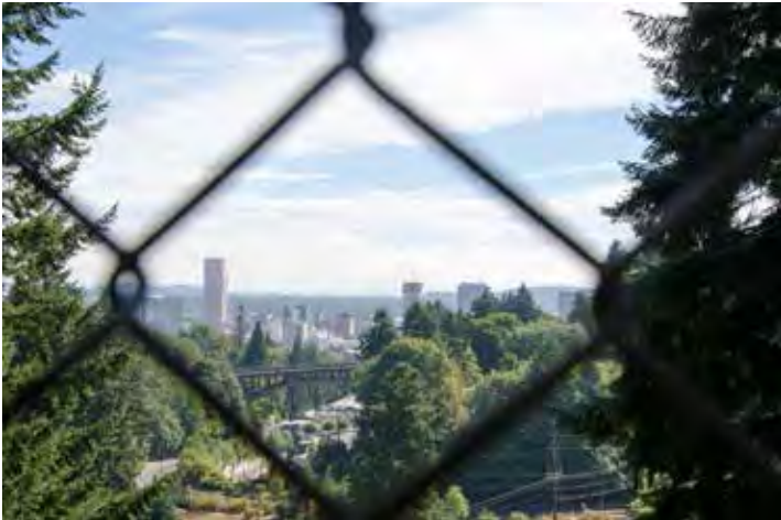
Vista Avenue Viaduct from SW Sherwood Boulevard
