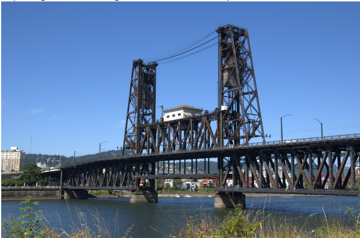
View of Steel Bridge as the primary focal feature.
