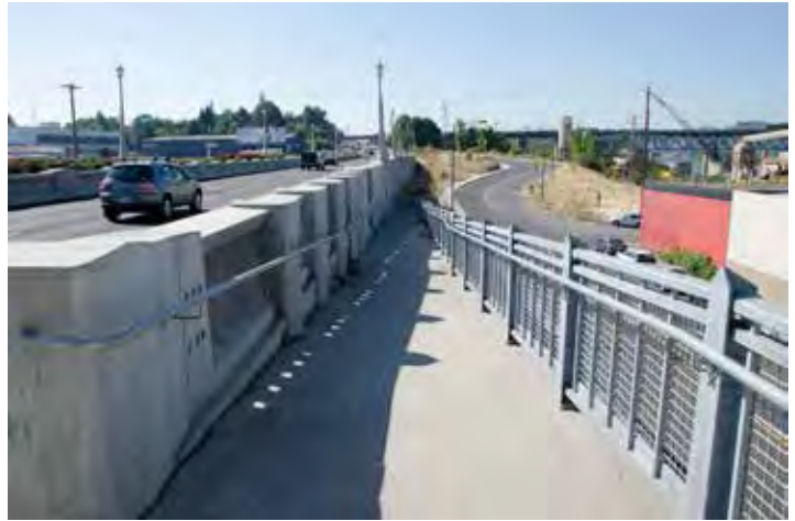
Ramp leading up to viewpoint at MLK Viaduct above SE Division Place
