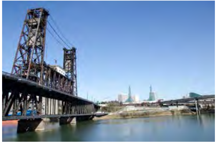
View from Greenway Trail south of Steel Bridge
