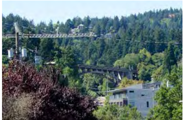
Vista Avenue Viaduct from SW Jefferson Street and SW 14th Avenue
