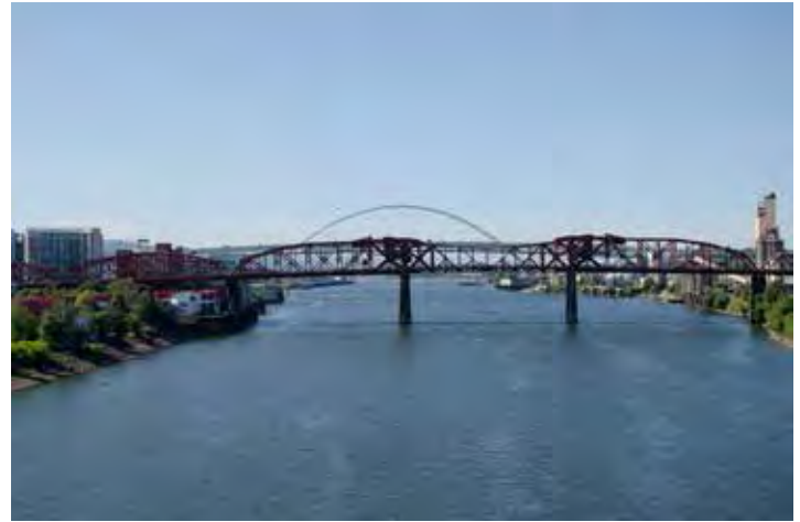
View from Steel Bridge north side center
