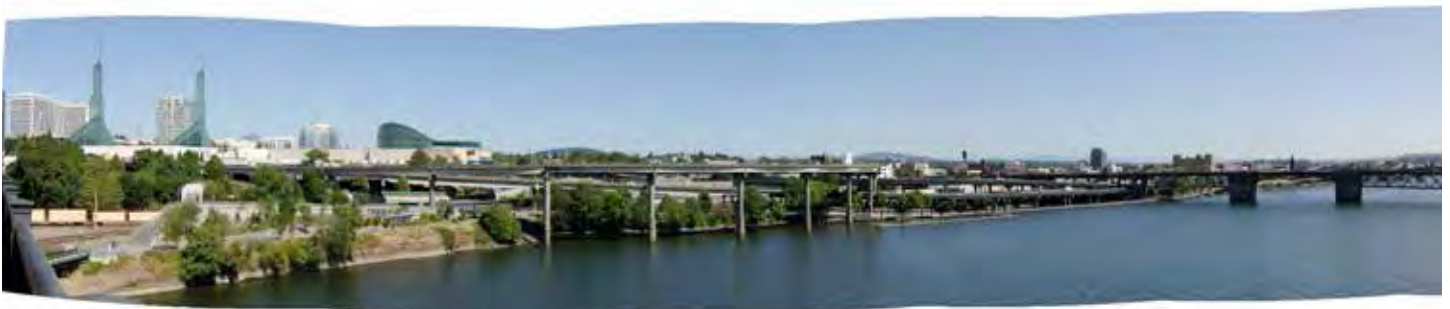
View from Steel Bridge upper deck, south side center
