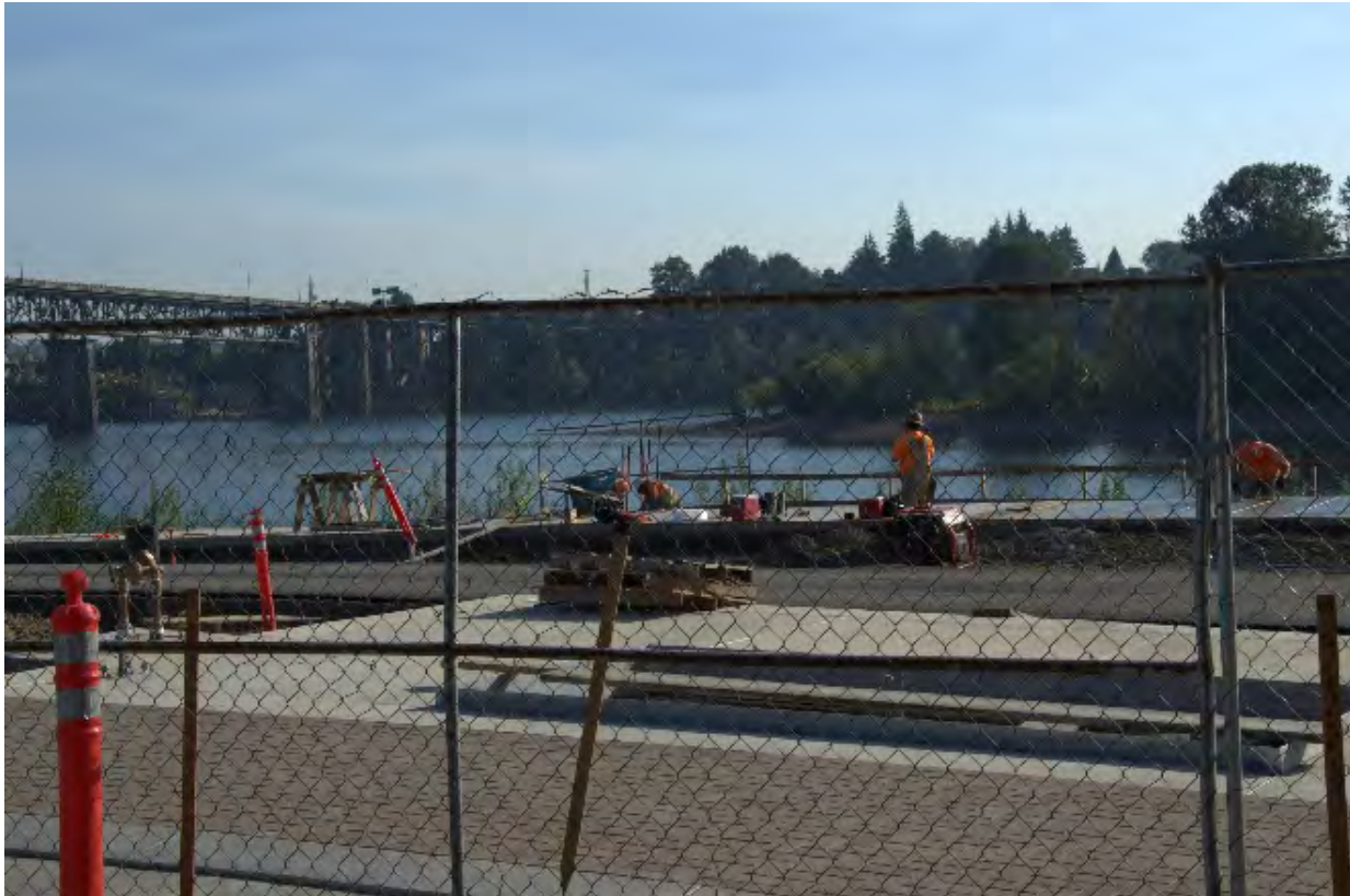
Example: Greenway Trail construction fencing
