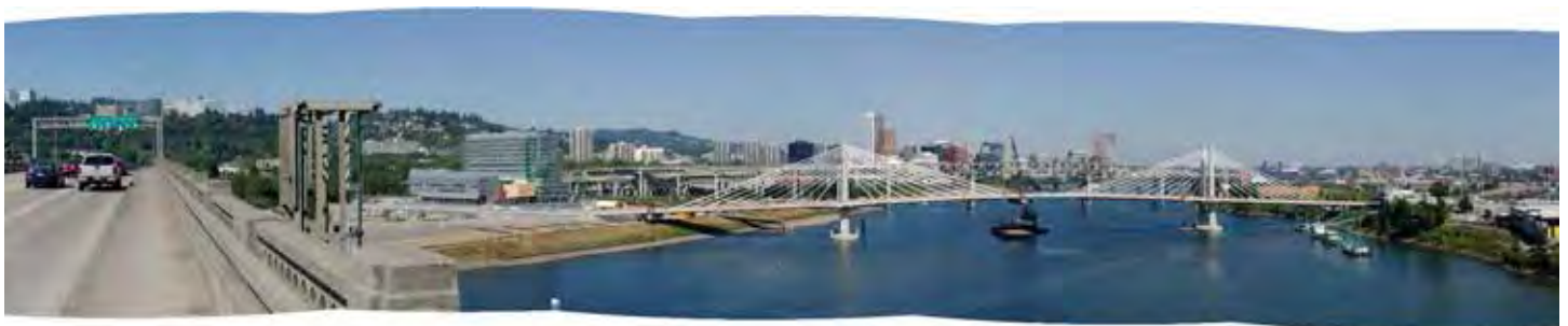
View from Ross Island Bridge north side center, looking north
