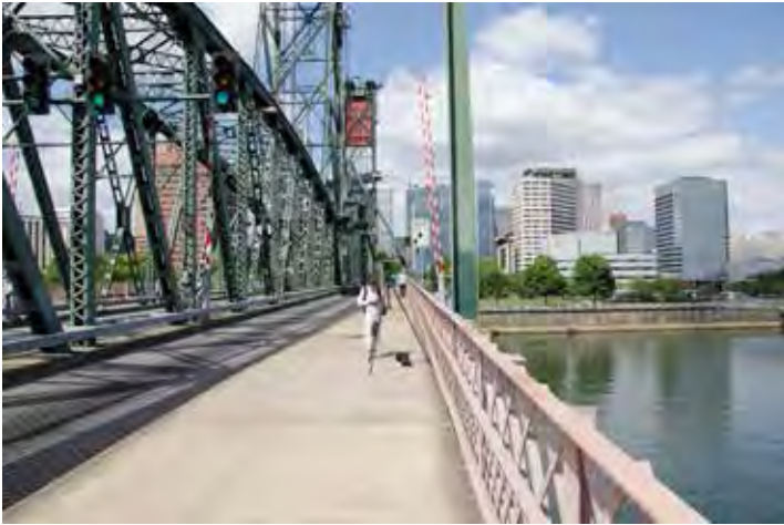
Viewpoint on Hawthorne Bridge north side center
