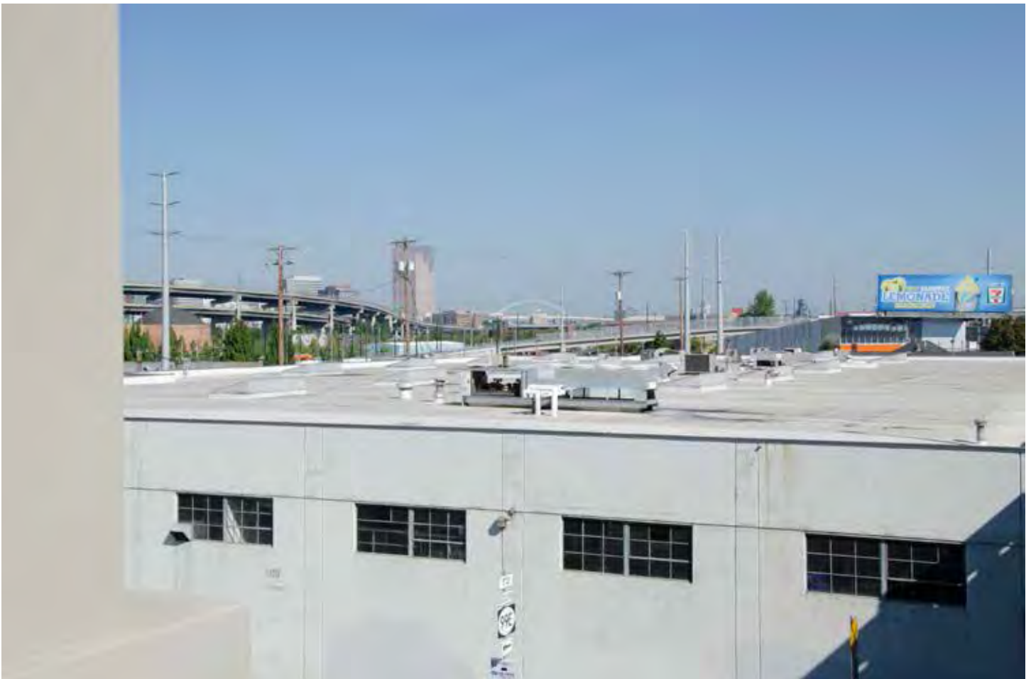
View from MLK Viaduct above SE Division Place, looking north
