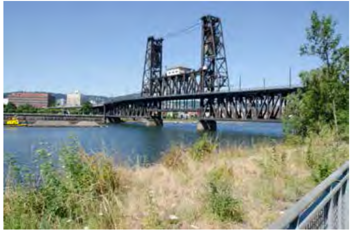
View of Steel Bridge from Eastbank Esplanade south of Steel Bridge
