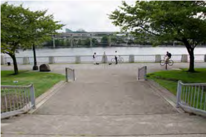
Viewpoint along Greenway Trail at stairs near NW Everett Street
