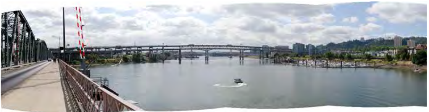
View from Hawthorne Bridge south side center
