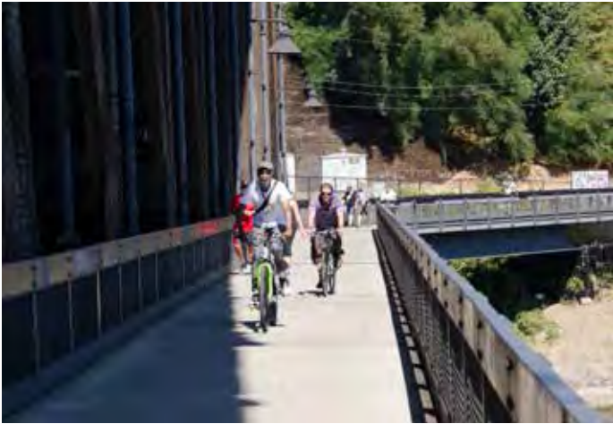
Viewpoint along Steel Bridge lower deck bike/pedestrian path
