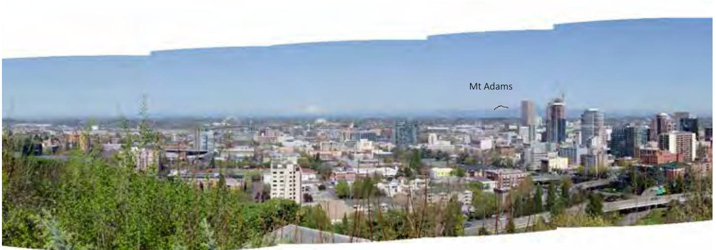
View from SW Upper Hall Street
