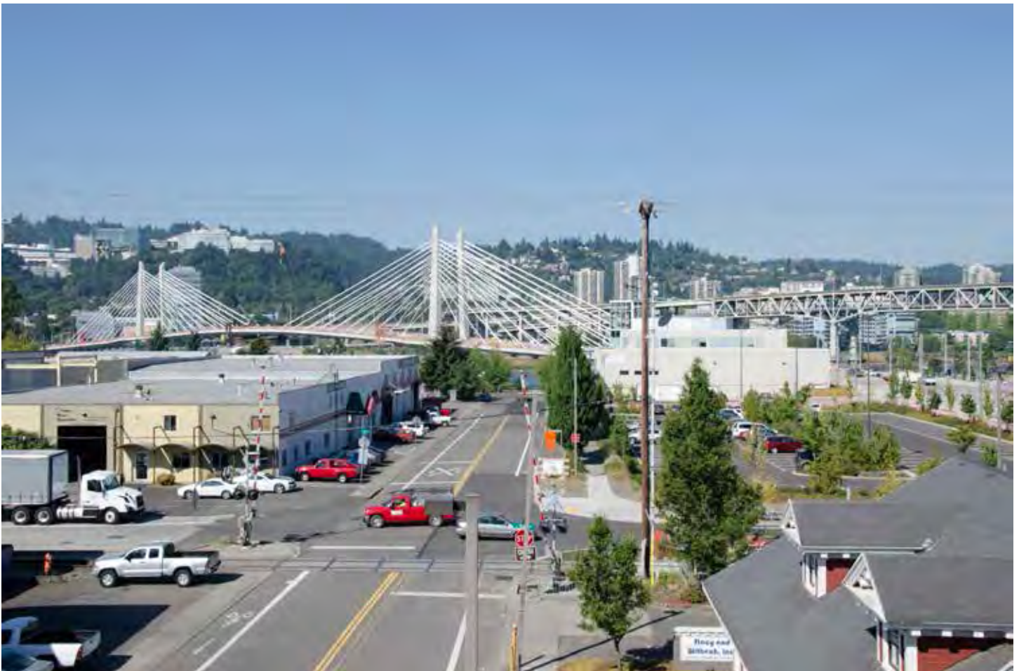
View from MLK Viaduct above SE Caruthers Street
