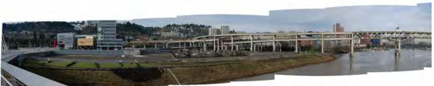
View from Tilikum Crossing, north side, west bump-out
