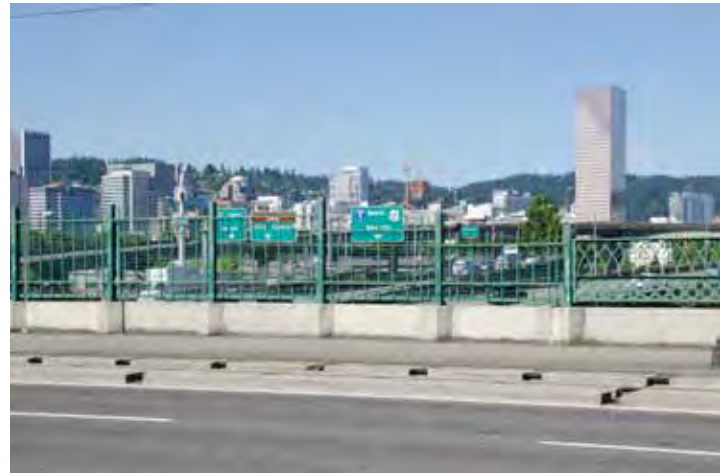
View from NE MLK Jr Boulevard and I-84 overpass
