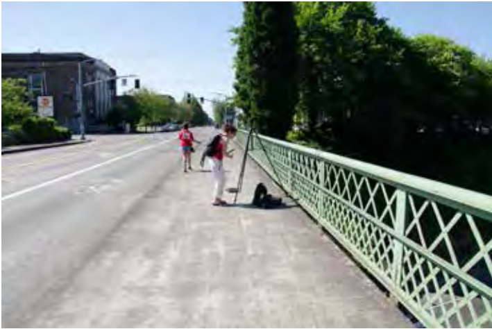
Viewpoint at NE 12th Avenue and I-84 overpass
