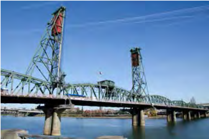
The Hawthorne Bridge from the Greenway Trail (west)
