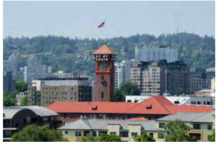
View of Union Station from Broadway Bridge south side center
