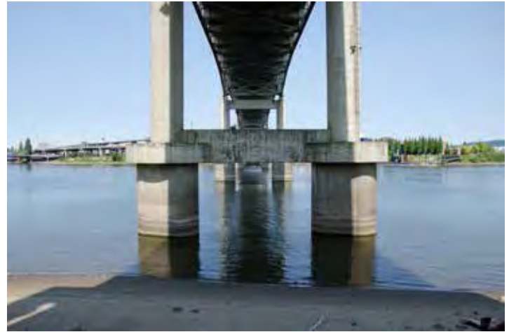
View from Greenway Trail under Marquam Bridge
