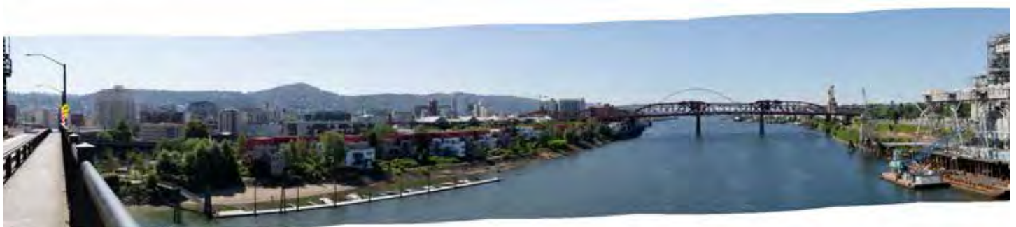
View from Steel Bridge north side center
