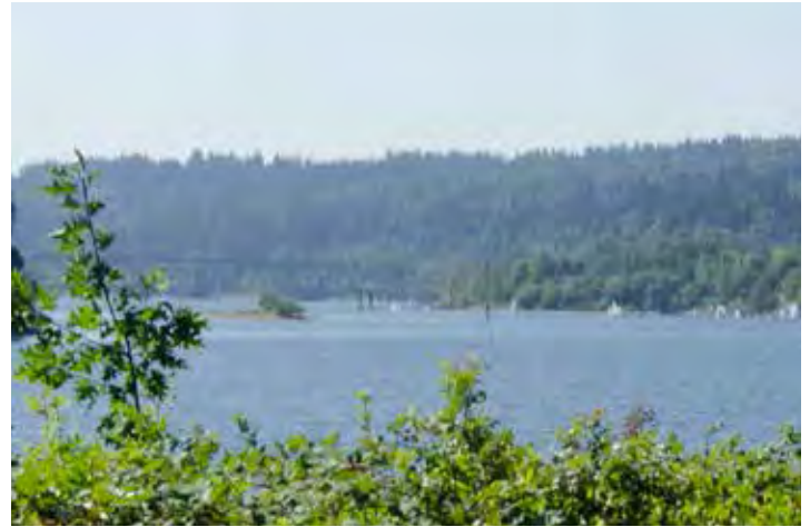
View of Sellwood Bridge from Greenway Trail at SW Bancroft Street
