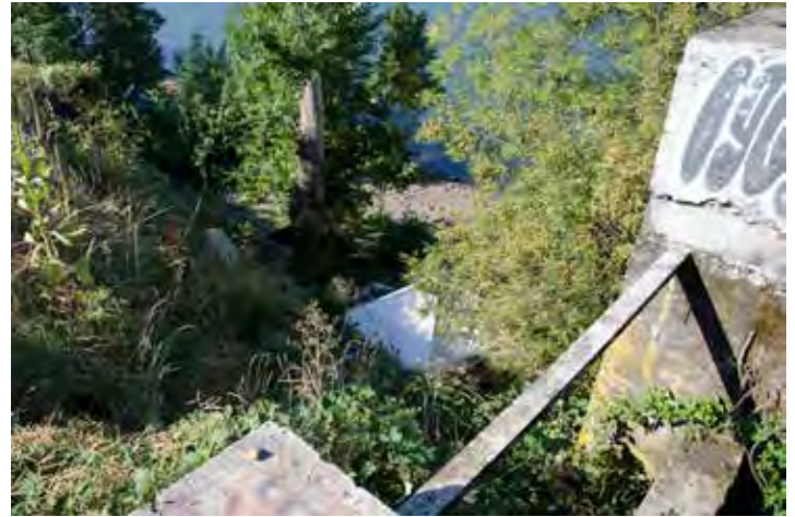
Viewpoint along Springwater Corridor between SE Franklin and Haig Streets
