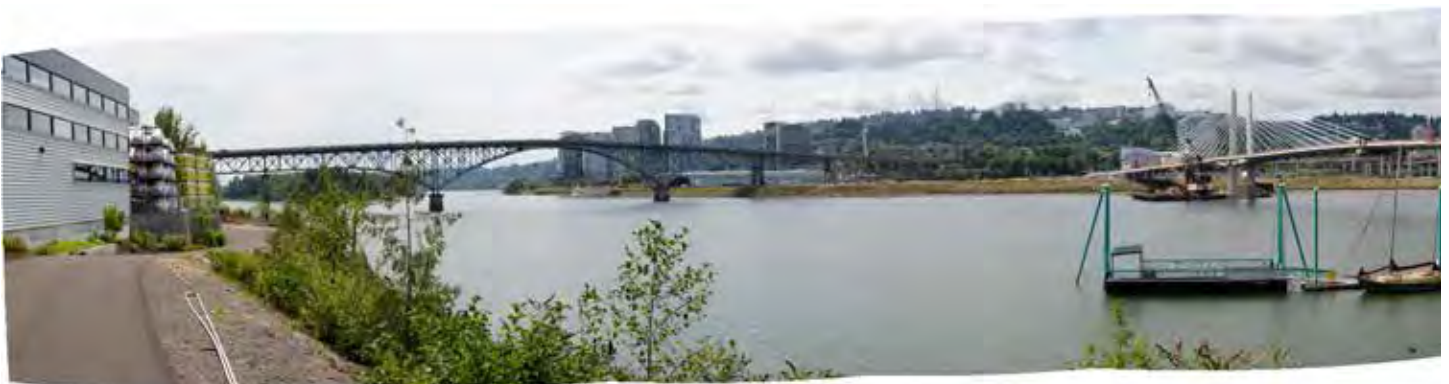
View from Greenway Trail (east) between SE Division Place and SE Ivon Street
