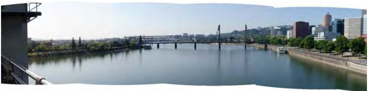
View from Morrison Bridge south side, west bump-out
