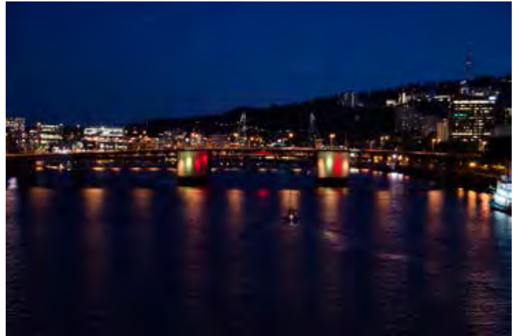
The Morrison Bridge from the Burnside Bridge at night
