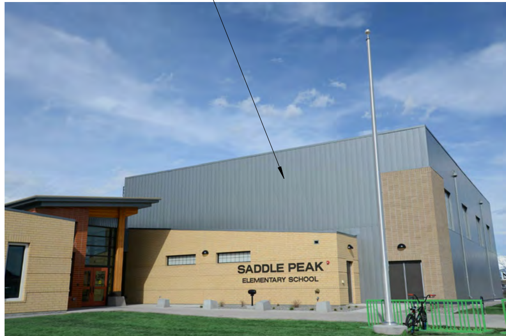
METAL PANEL - 12" WIDE FLUSH INTERLOCK
