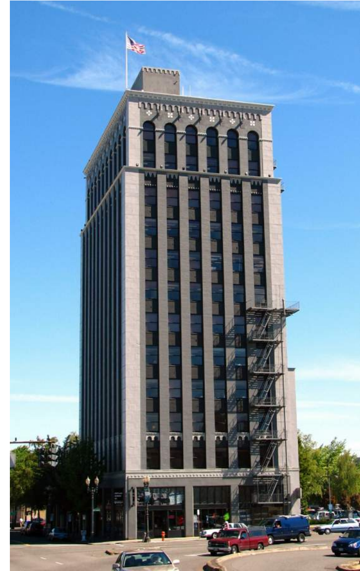
WEATHERLY BUILDING PORTLAND
