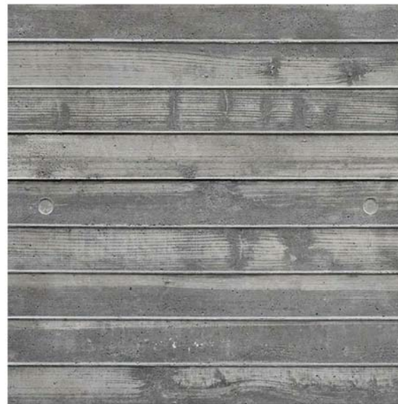
1 BOARDFORM CAST-IN-PLACE CONCRETE
