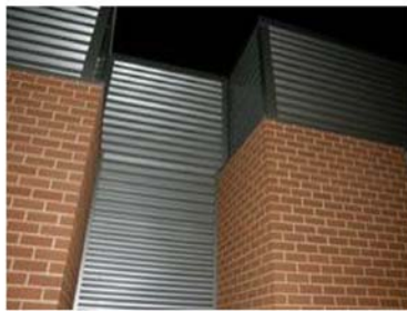
BRICK TO METAL EXAMPLE OF SIDING TRANSITION
