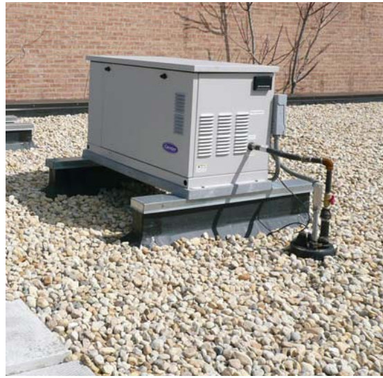
Example: Roof Mounted Generator
