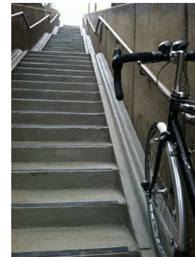
Concept Images of Concrete Stair/Bike Ramp To allow residents access to the second level bike room from SW 4th Avenue.
