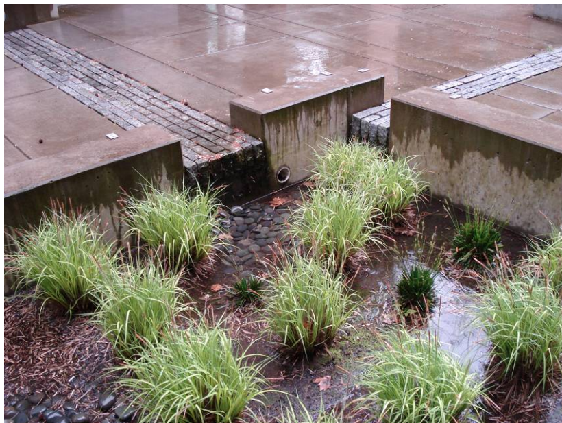
Exhibit 2-19: Epler Hall Planter. See Appendix G.1 , SW-130, for typical private property planter detail and Appendix G.3 , SW-310 through SW-313, for typical Green Street planter details.
