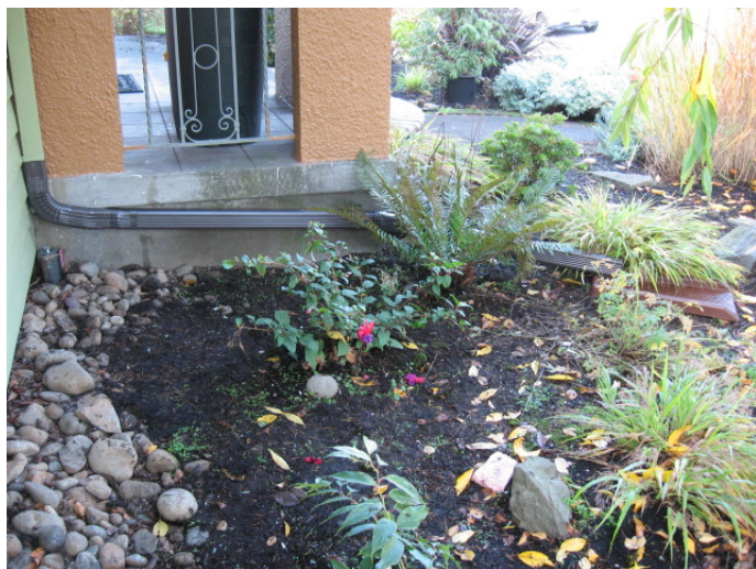
Exhibit 2-10. Disconnected downspout.
