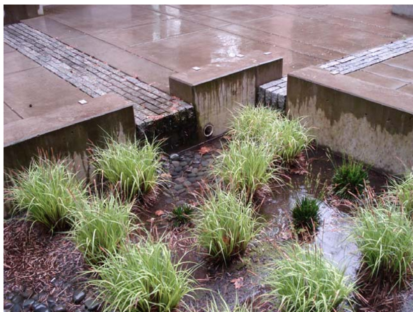
Exhibit 2-16: Epler Hall Planter. See Appendix G.1 SW-130 for typical private property planter detail and Appendix G.3 SW-310 through SW-313 for typical Green Street planter details.
