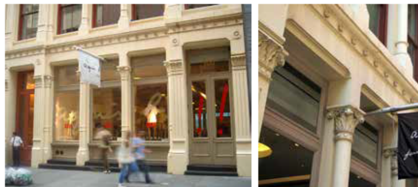
The details used in this 1998 reconstruction project in SoHo were designed based on historical photographs and an adjacent sister building.
