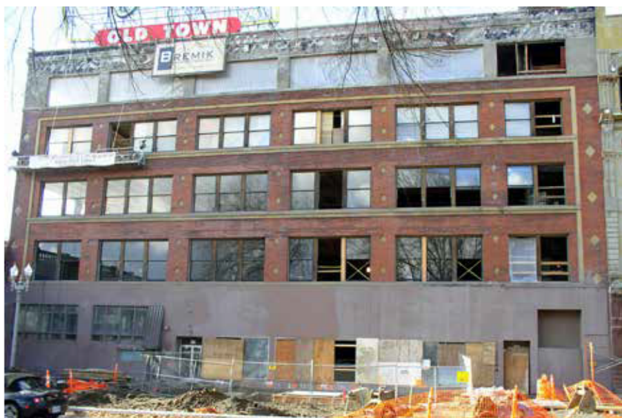
The wood windows at the White Stag/Hirsch Weis Building were rehabilitated rather than replaced.
