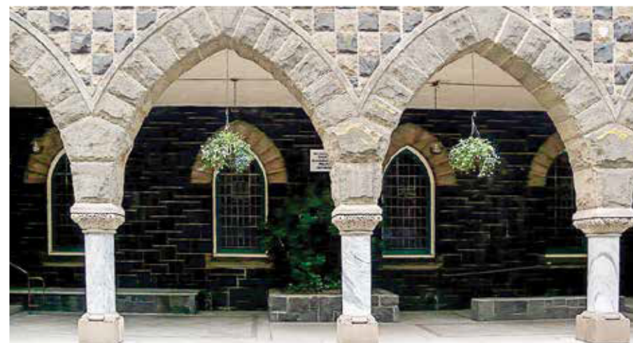
The upgrade of the First Congregational Church (1126 SW Park Ave) hid new structural members inside the columns so as not to disrupt the historic character of the building.
