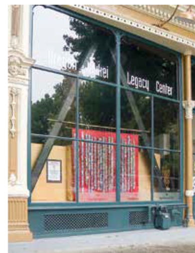
By locating the steel cross bracing well behind the building façade, its visual impact is greatly reduced.
