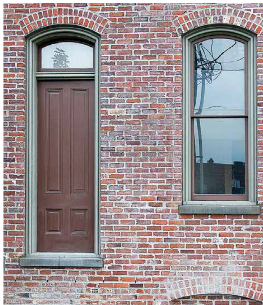
At the West Block located at 701 SE Grand Ave, a historic door was fixed in place rather than bricking it over, which allowed the original character of the building to be retained even though the door is no longer used for egress.
