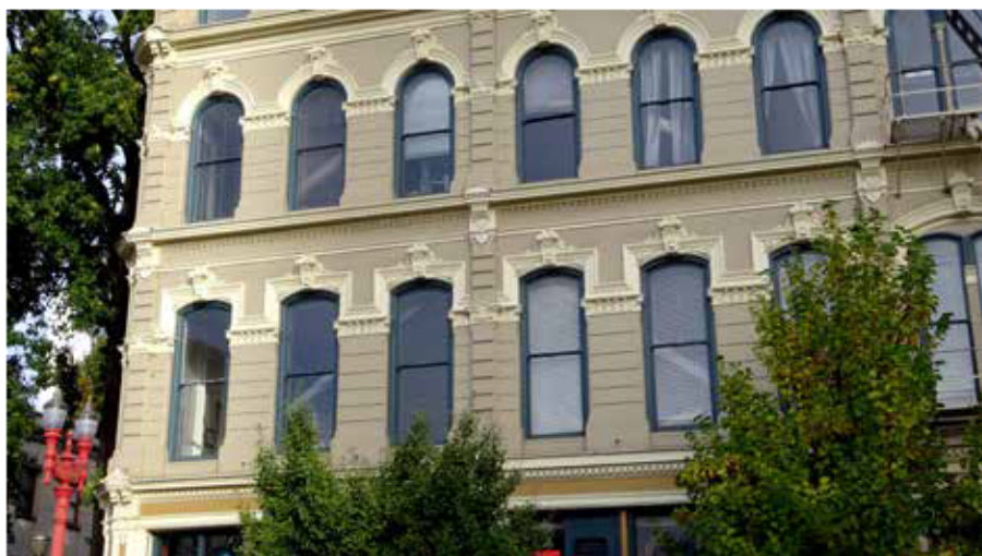
The renovation of the Merchant Block involved repairing all of the original wood windows.
