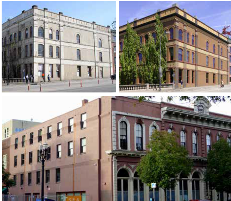
The Skidmore Block and the Smith Block are examples of rehabilitation projects where new window openings were introduced on secondary elevations. The new window placement respects the composition of the whole wall and the new sashes are of a material and level of quality that is compatible with the historic windows.
