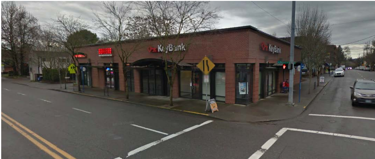
Figure 4 - Tacoma Site Frontage Along SE Tacoma Street
