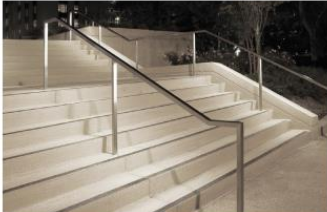
B CONCRETE STEPS W/ SS RAILINGS
