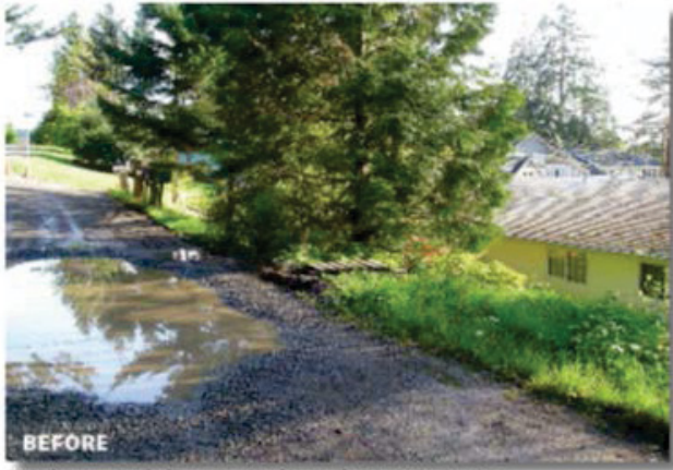
SW 28th Avenue South of Texas Street Looking North: Prior to Construction
