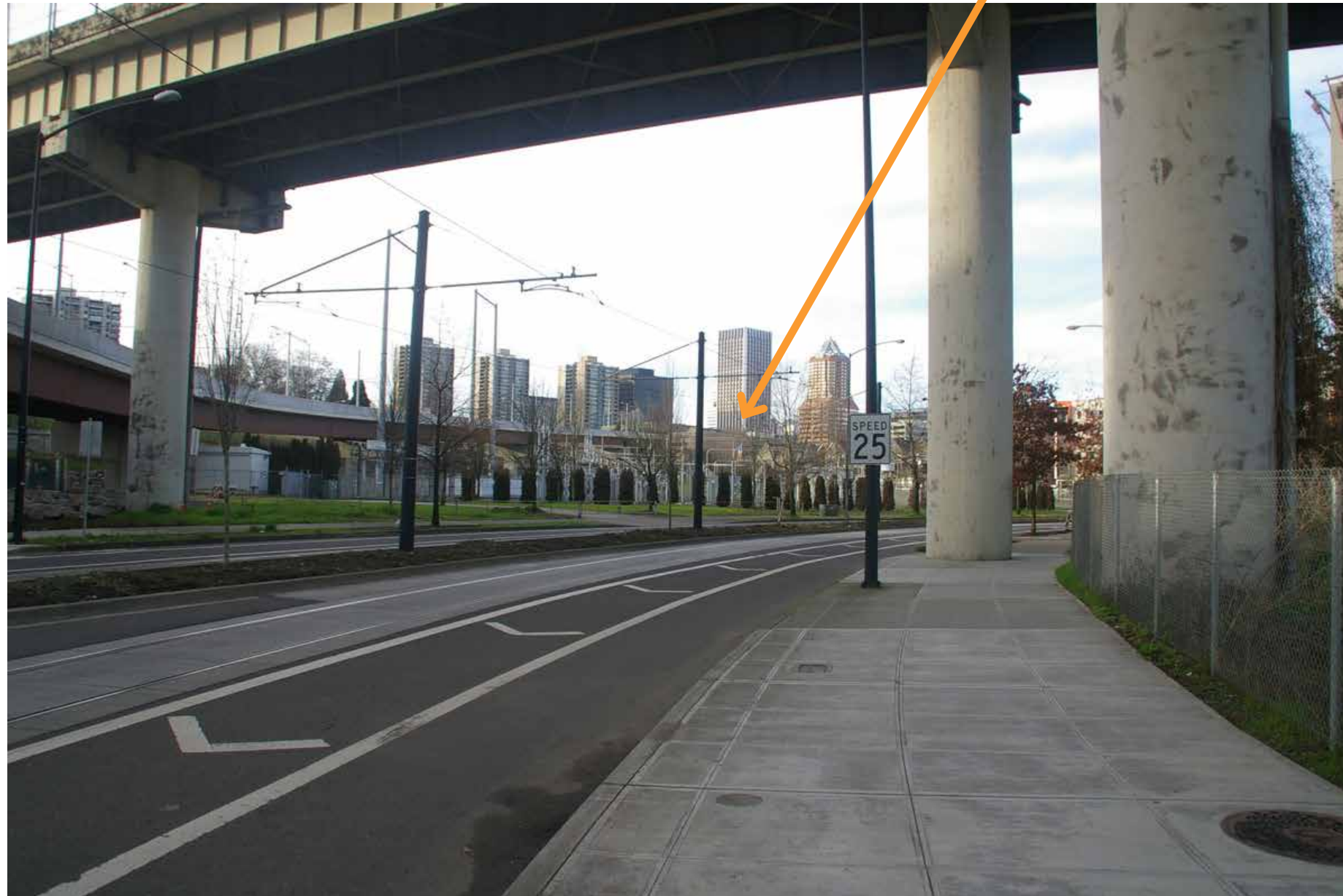
VIEW FROM MOODY AVE LOOKING NORTH
