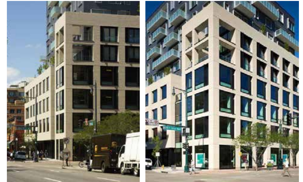
DEEP RECESSED WINDOWS WITH METAL SILL
