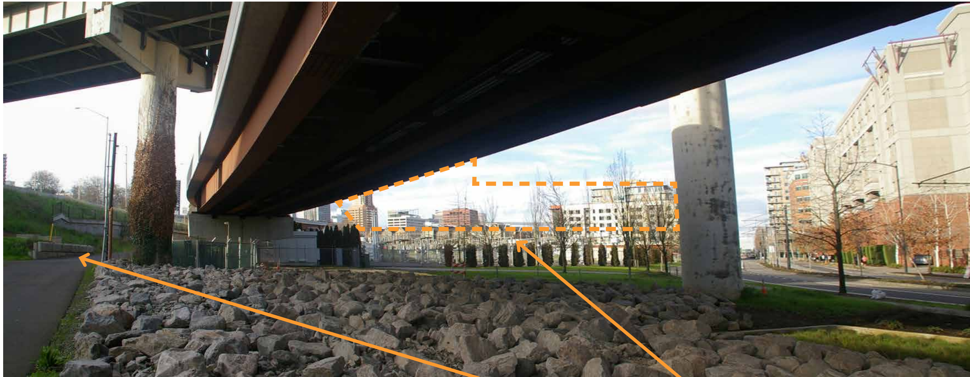
VIEW FROM MOODY AVE LOOKING NORTH FROM SOUTHWEST PORTION OF BIKE BATH
