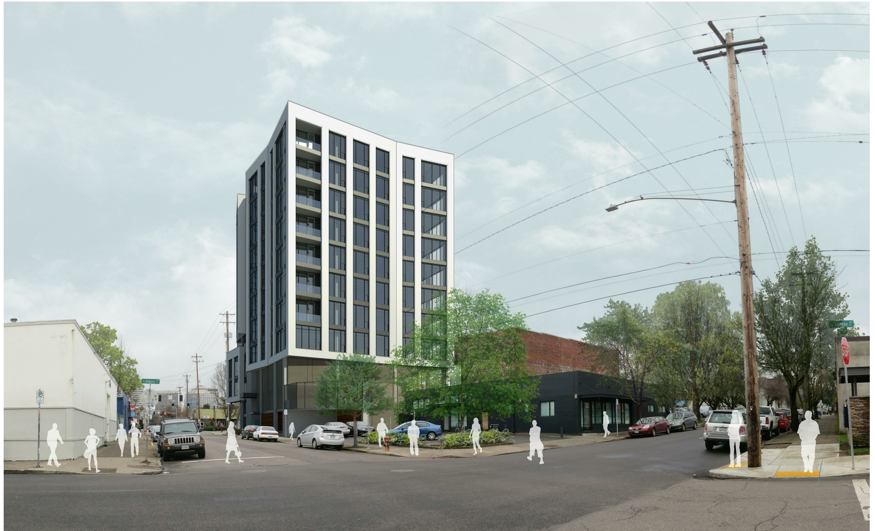
VIEW FROM THE SOUTHWEST - SE ANKENY STREET & SE 7TH AVENUE
