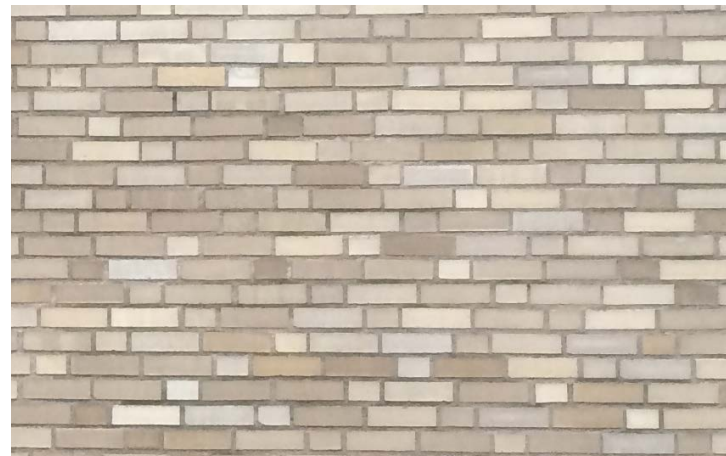
existing stott center brick bond pattern
