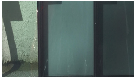
VISION SPANDREL SPANDREL #2 #1
