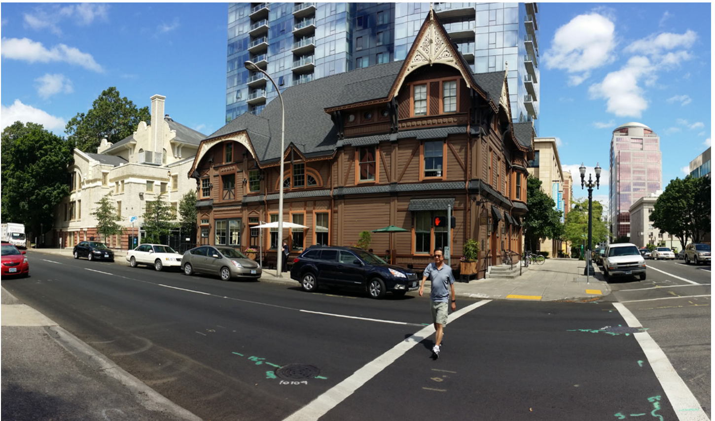
View from site looking north at intersection of SW Broadway and SW Columbia St.
