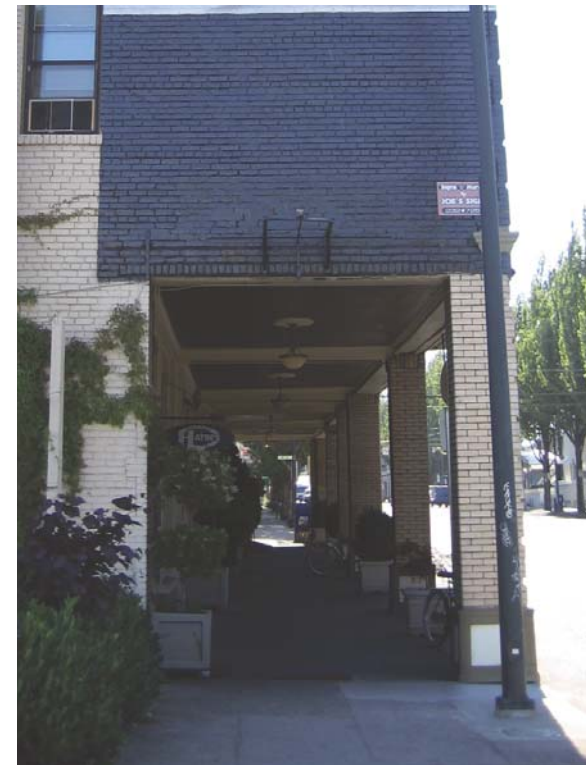
Burnside Arcade Condition
