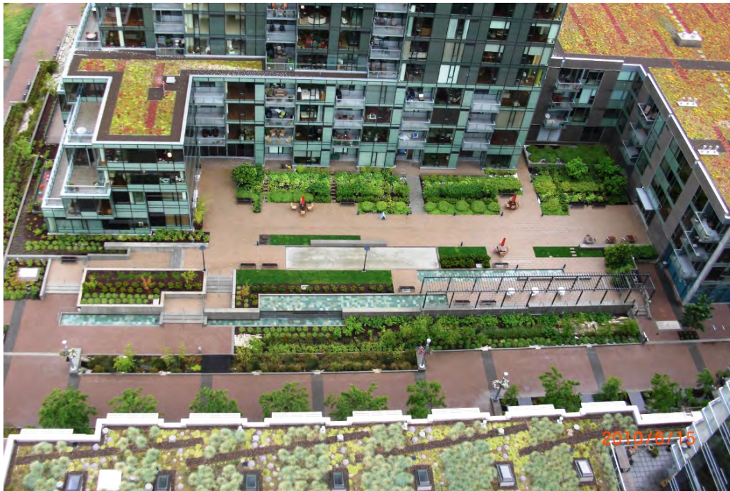
Example of a range of landscaping approaches integrated into urban development, including ecoroofs, raised landscaped areas, and stormwater planters.
