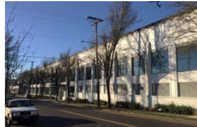
2 - PROPERTY TO THE WEST - JANTZEN BUILDING
