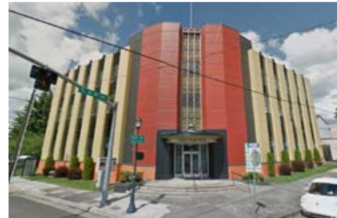
2 - SANDY PLAZA BUILDING
