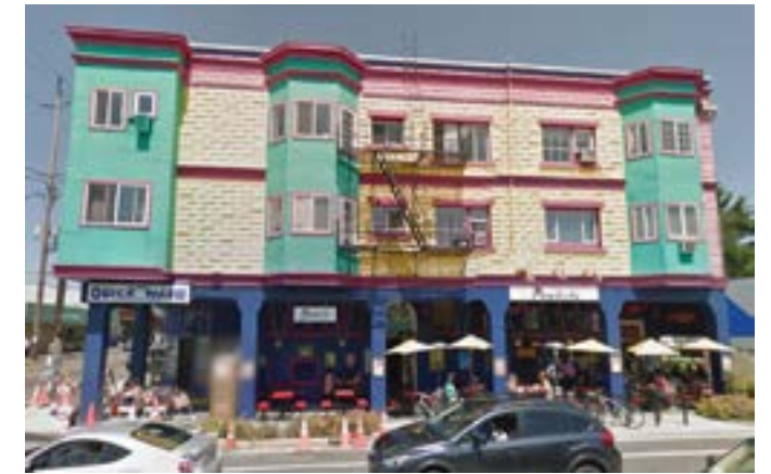
4 - NE GLISAN ST AND NE 29TH AVE
