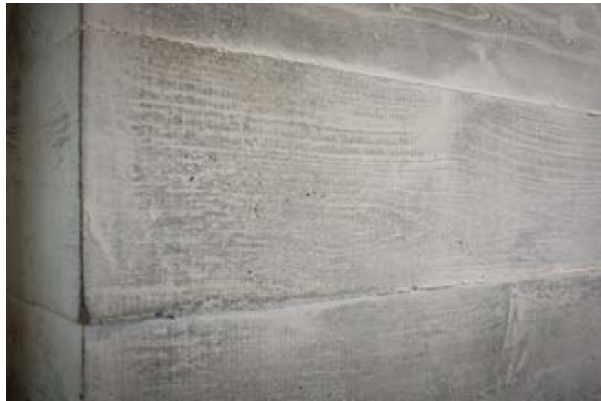
BOARD FORM CONCRETE - JOINT
