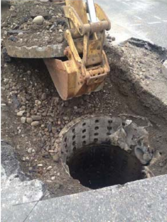
Previously paved-over UIC ADV573 being uncovered
