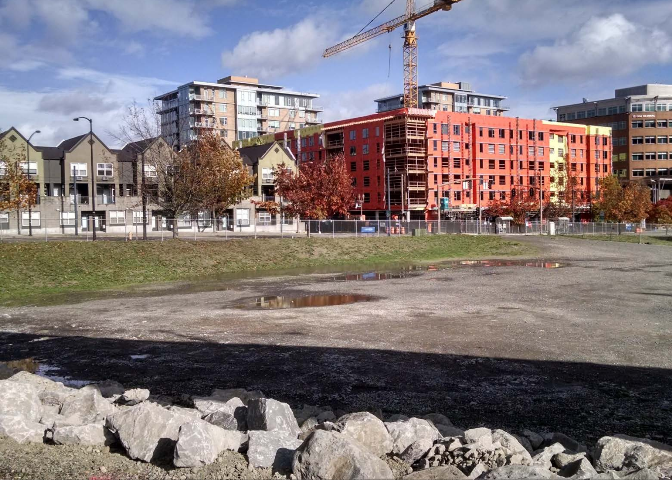
View to northeast
