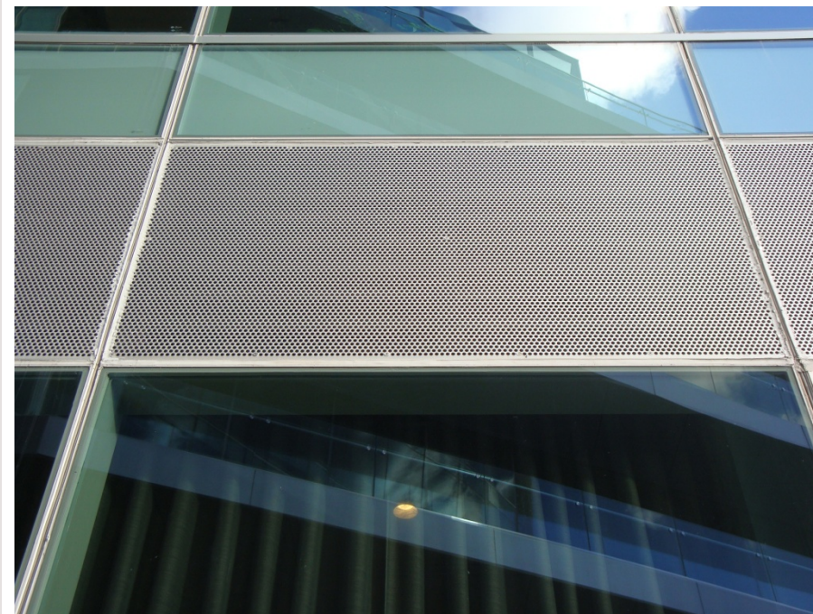
Close-up with louver behind (typical)
