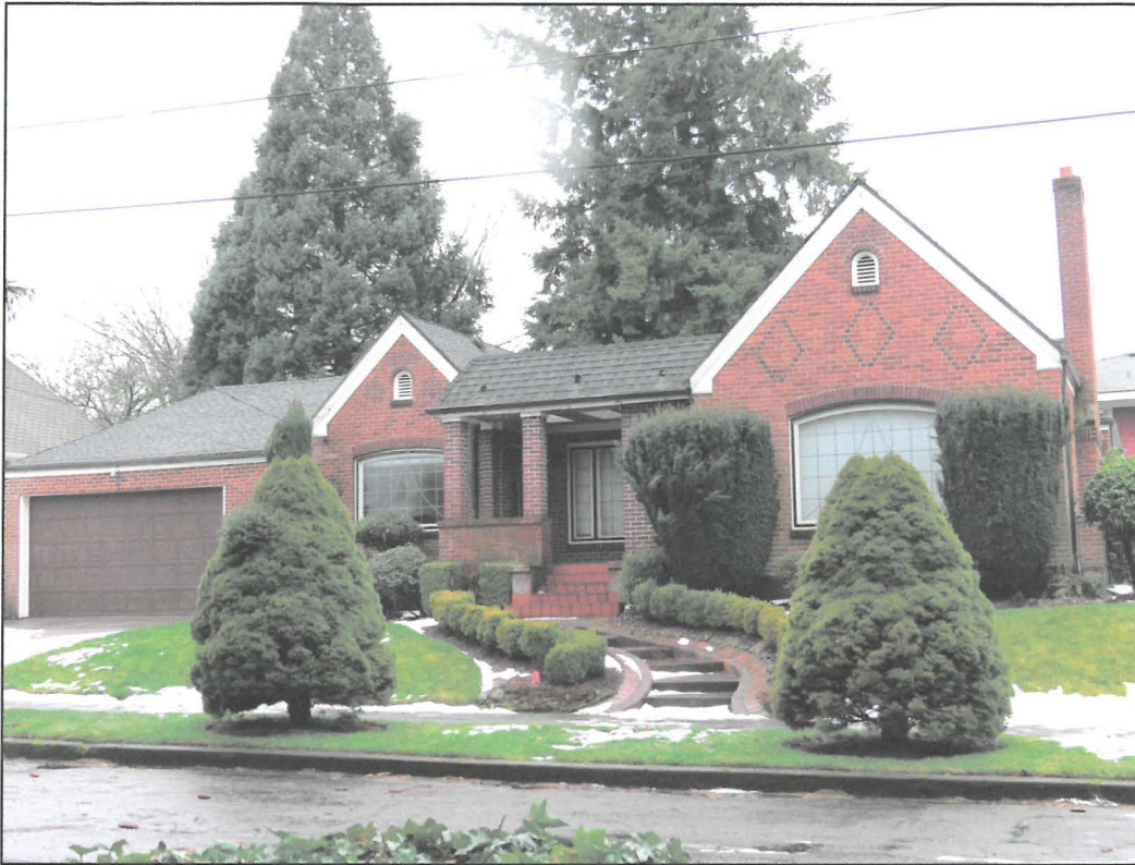
Bought for $725,000 to be demolished 3587 square feet House in excellent condition
