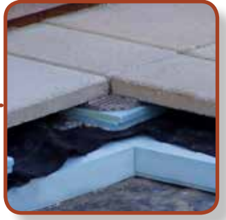
LEVEL 01 PATIOS CONCRETE PEDESTAL PAVERS
