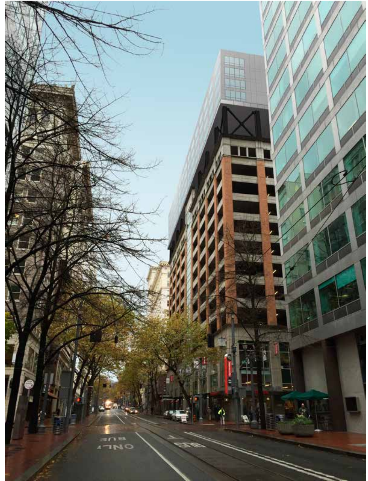
view from north
